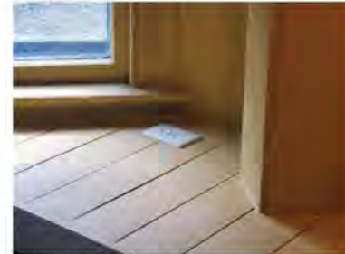
1st Floor East Bedroom
