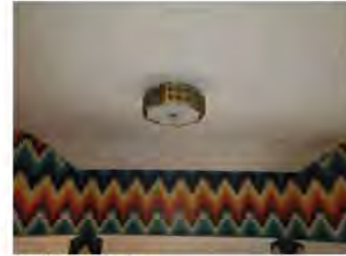
2nd Floor Stairs
