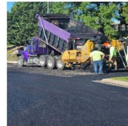
Plaza Paving Progress
