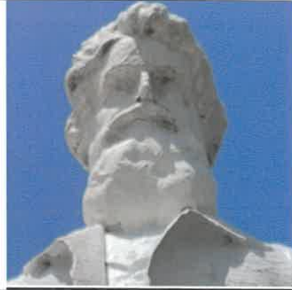
Marble is possibly covered in thick white paint.
