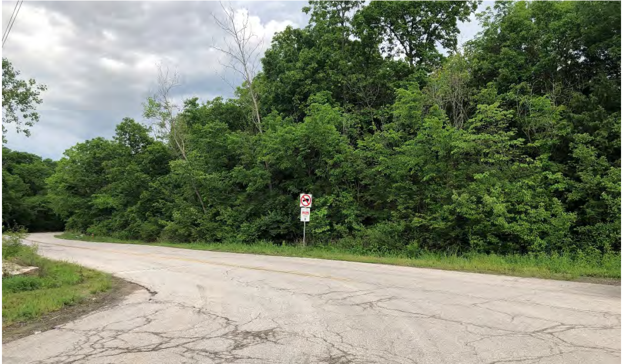
Figure 1. Site Photograph of 6601 Inland Drive looking northwest from South 65th Street (provided by Planning Staff).
