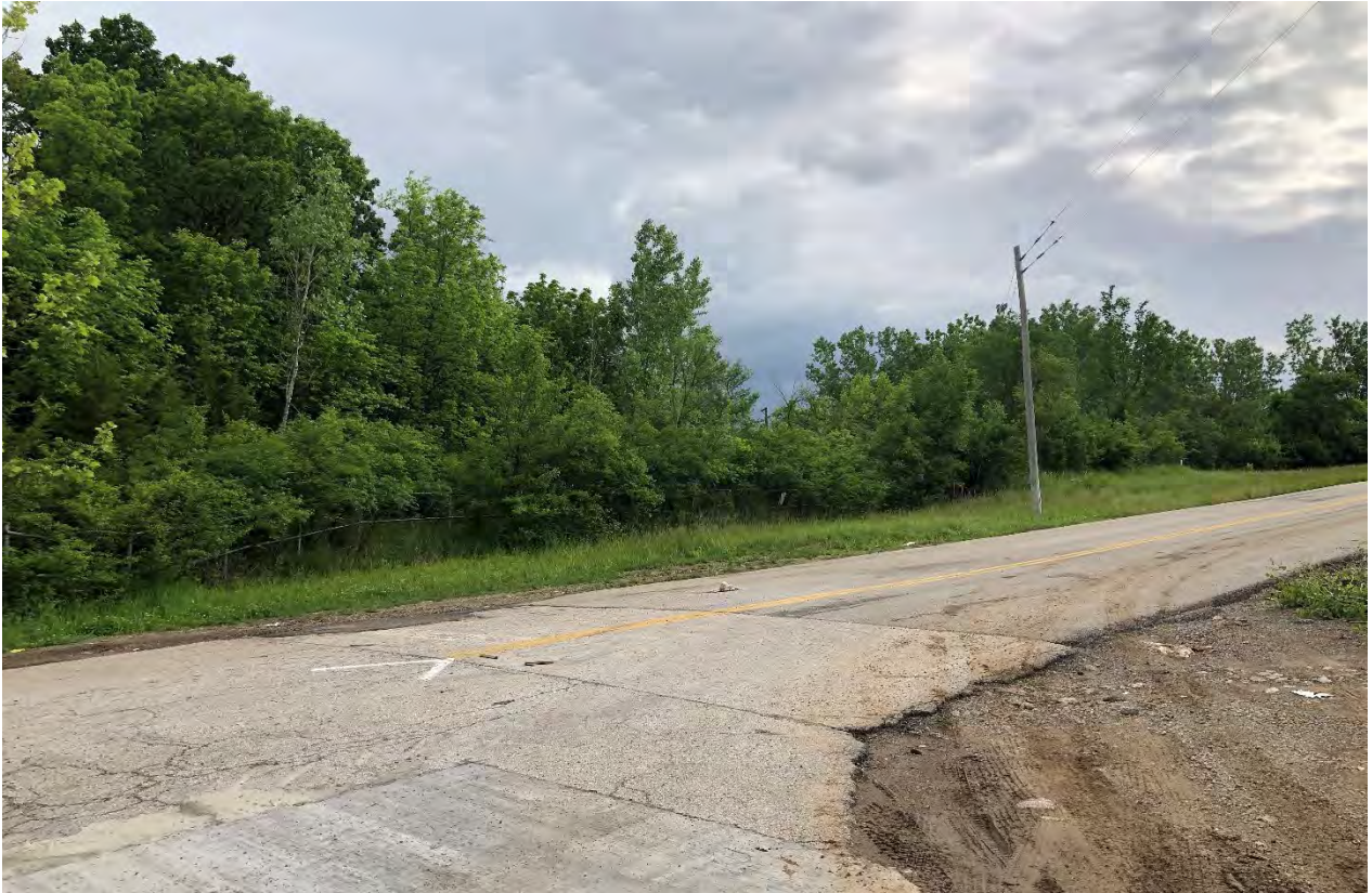
Figure 3. Site Photograph of 6601 Inland Drive looking northeast from South 65th Street (provided by Planning Staff).
