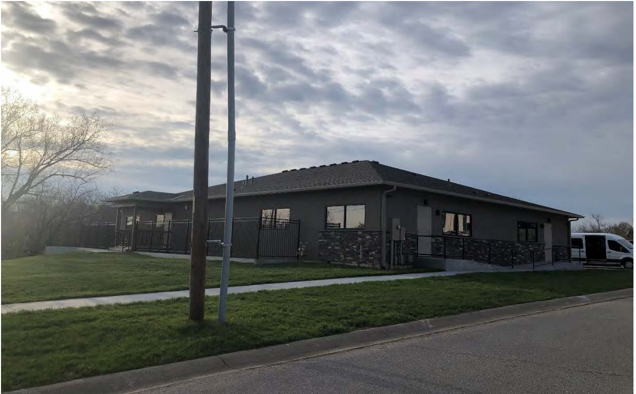
Figure 4. Site Photograph of 9151 Parallel Parkway looking southeast from the private drive (provided by Planning Staff).
