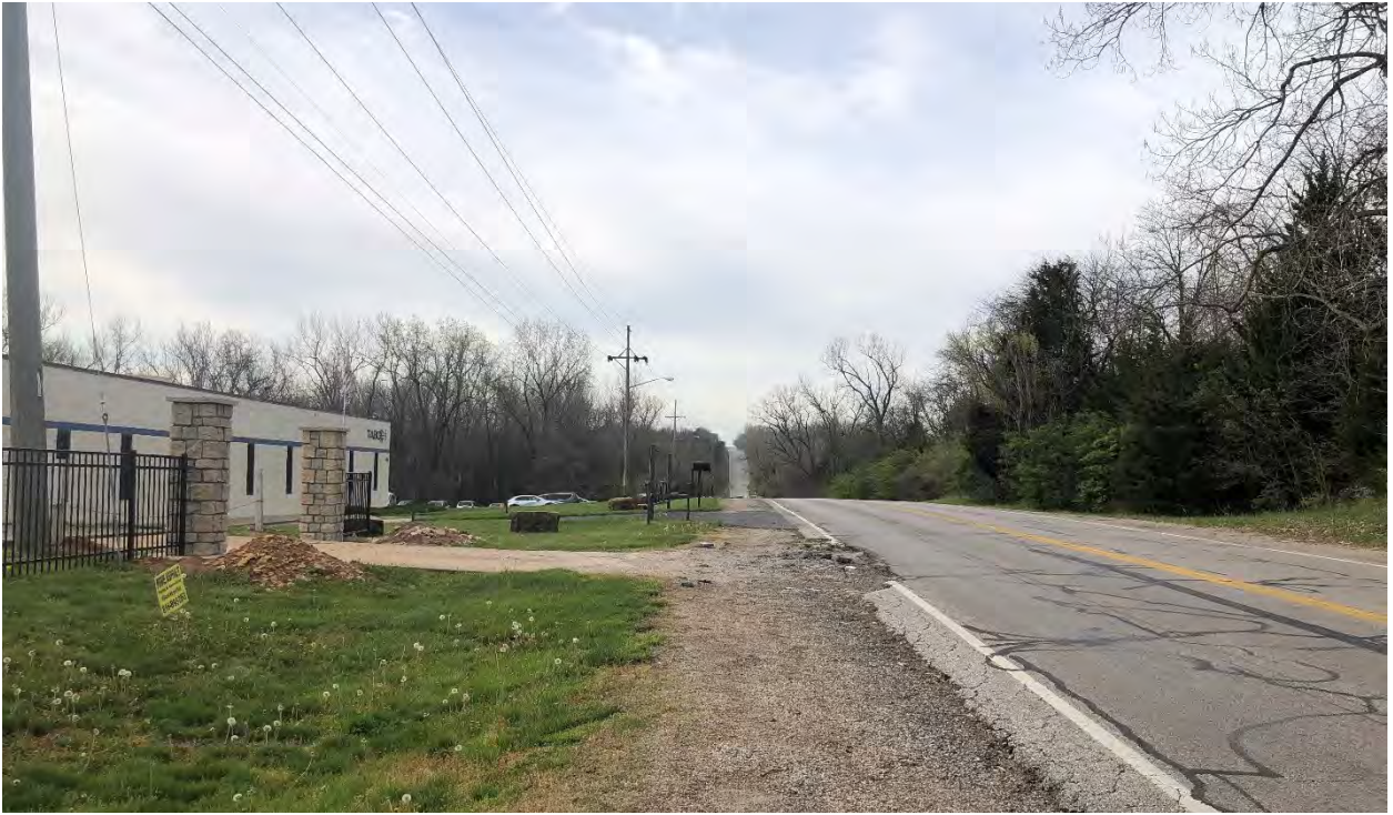
Figure 9. Site photograph looking south from South 59th Street at 1323 South 59th Street (provided by Planning Staff).
