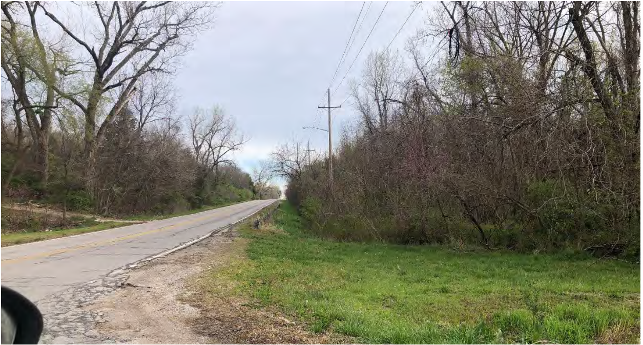
Figure 4. Site photograph looking north from Metropolitan Avenue at 1323 South 59 th Street (provided by Planning Staff).
