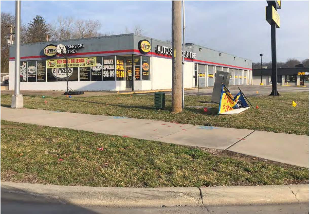
Figure 6. Site photograph of 7908 State Avenue looking northwest from State Avenue (provided by Planning Staff).
