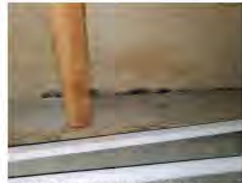
Basement (Behind Water Heater)
