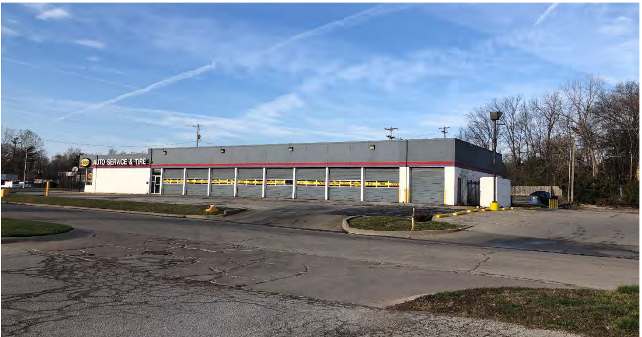
Figure 7. Site photograph of 7908 State Avenue looking southwest from North 98 th Street (provided by Planning Staff).
