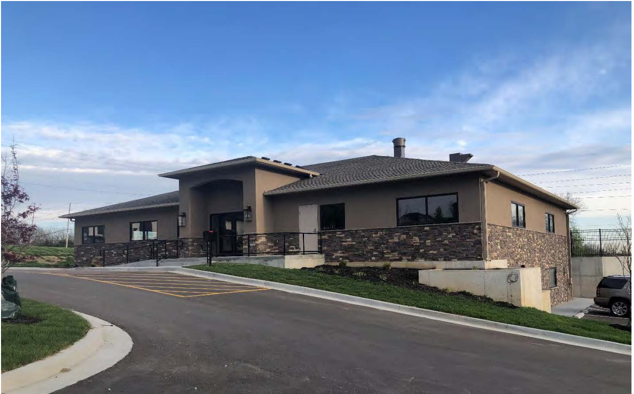
Figure 6. Site Photograph of 9151 Parallel Parkway looking northwest from the parking lot (provided by Planning Staff).
