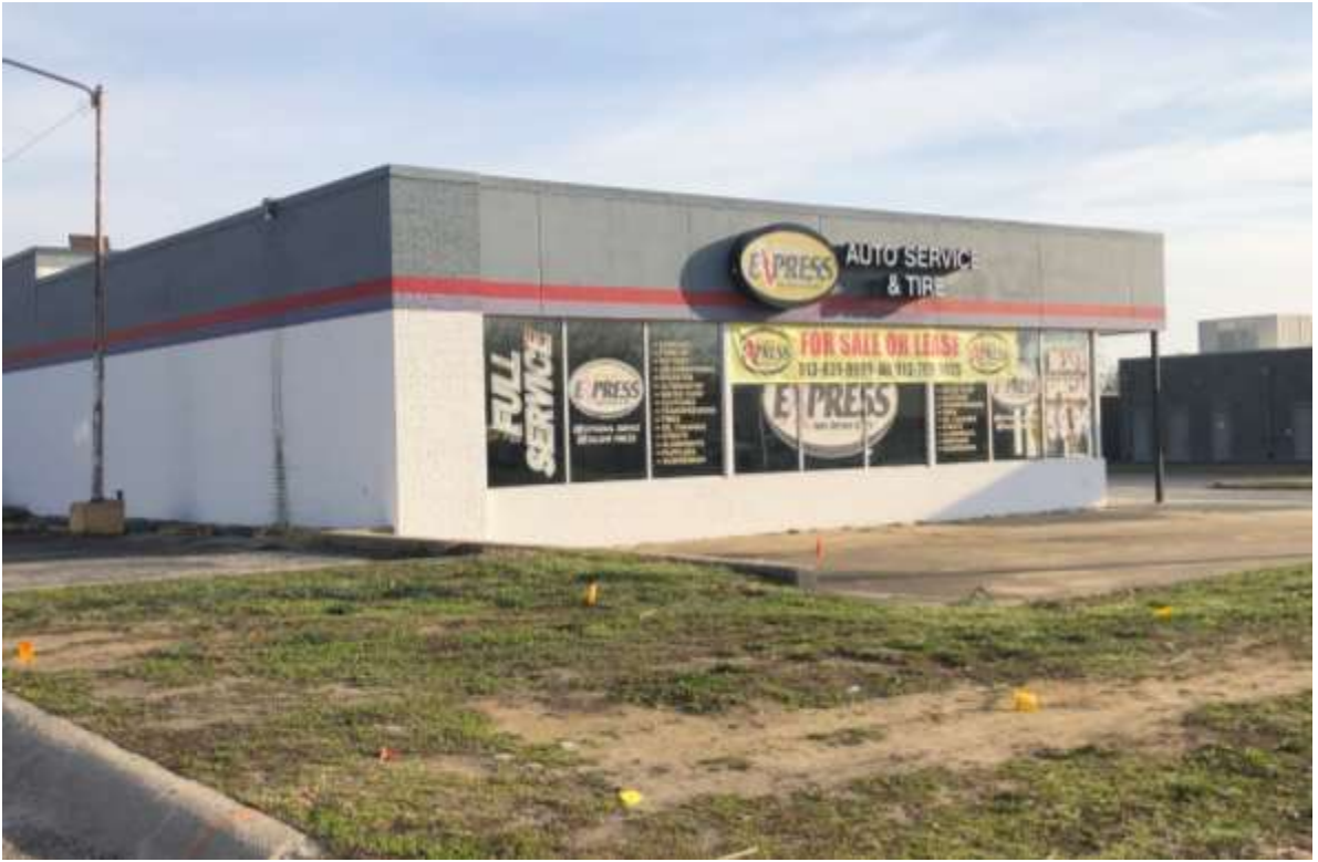
Figure 4. Site photograph of 7908 State Avenue looking northeast from State Avenue (provided by Planning Staff).
