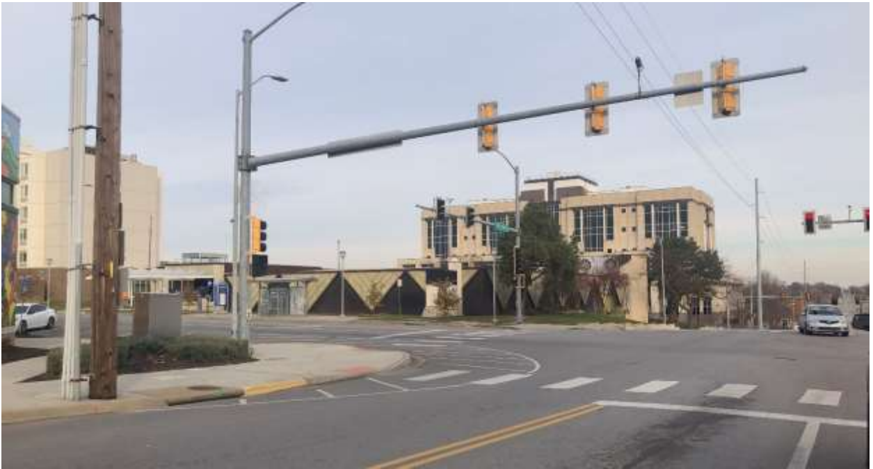
Figure 4. Site Photograph of the Reardon Civic Center from North 5 th Street looking northwest (provided by Planning Staff).
