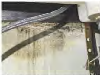
3065 1st Floor bathroom under sink
