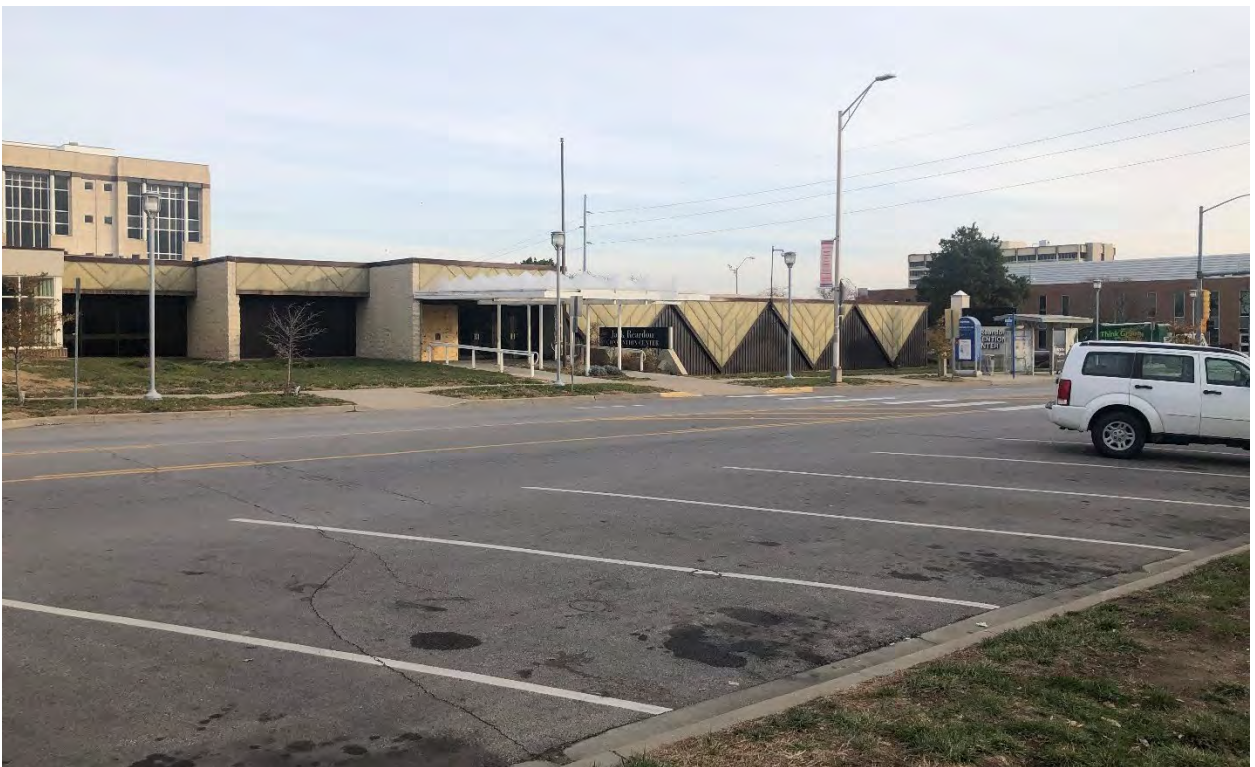
Figure 5. Site Photograph of the Reardon Civic Center from Minnesota Avenue looking northeast (provided by Planning Staff).
