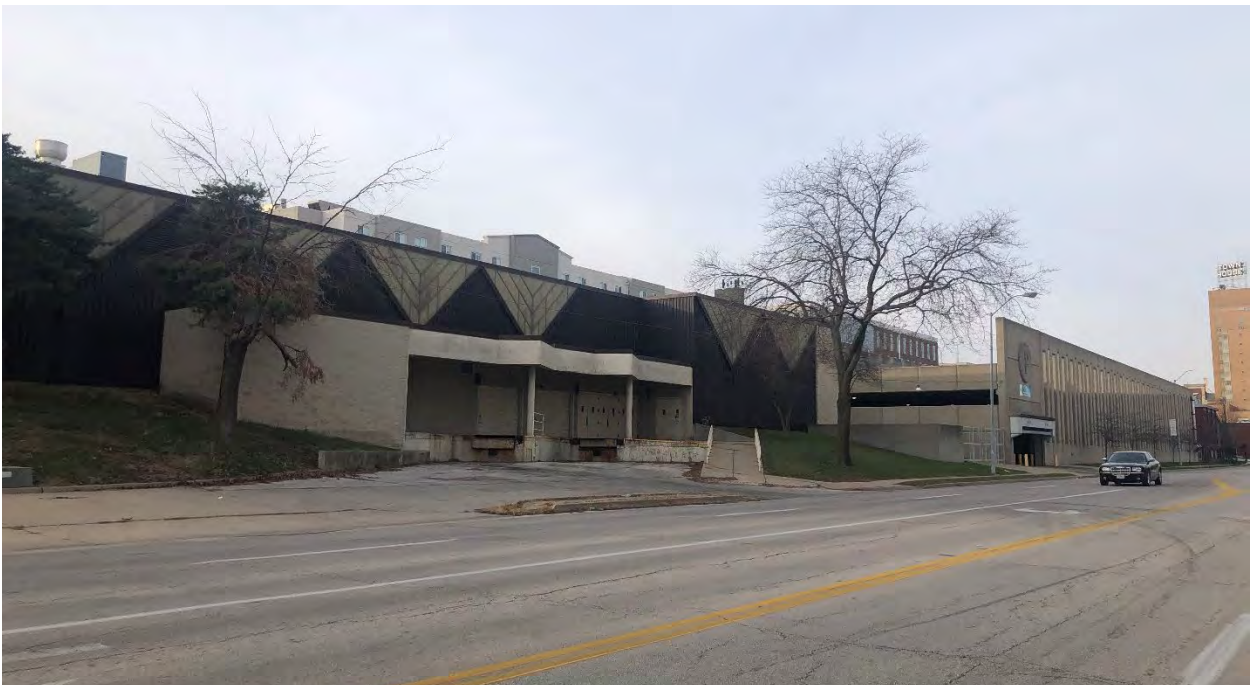
Figure 7. Site Photograph of the Reardon Civic Center from State Avenue looking southwest (provided by Planning Staff).
