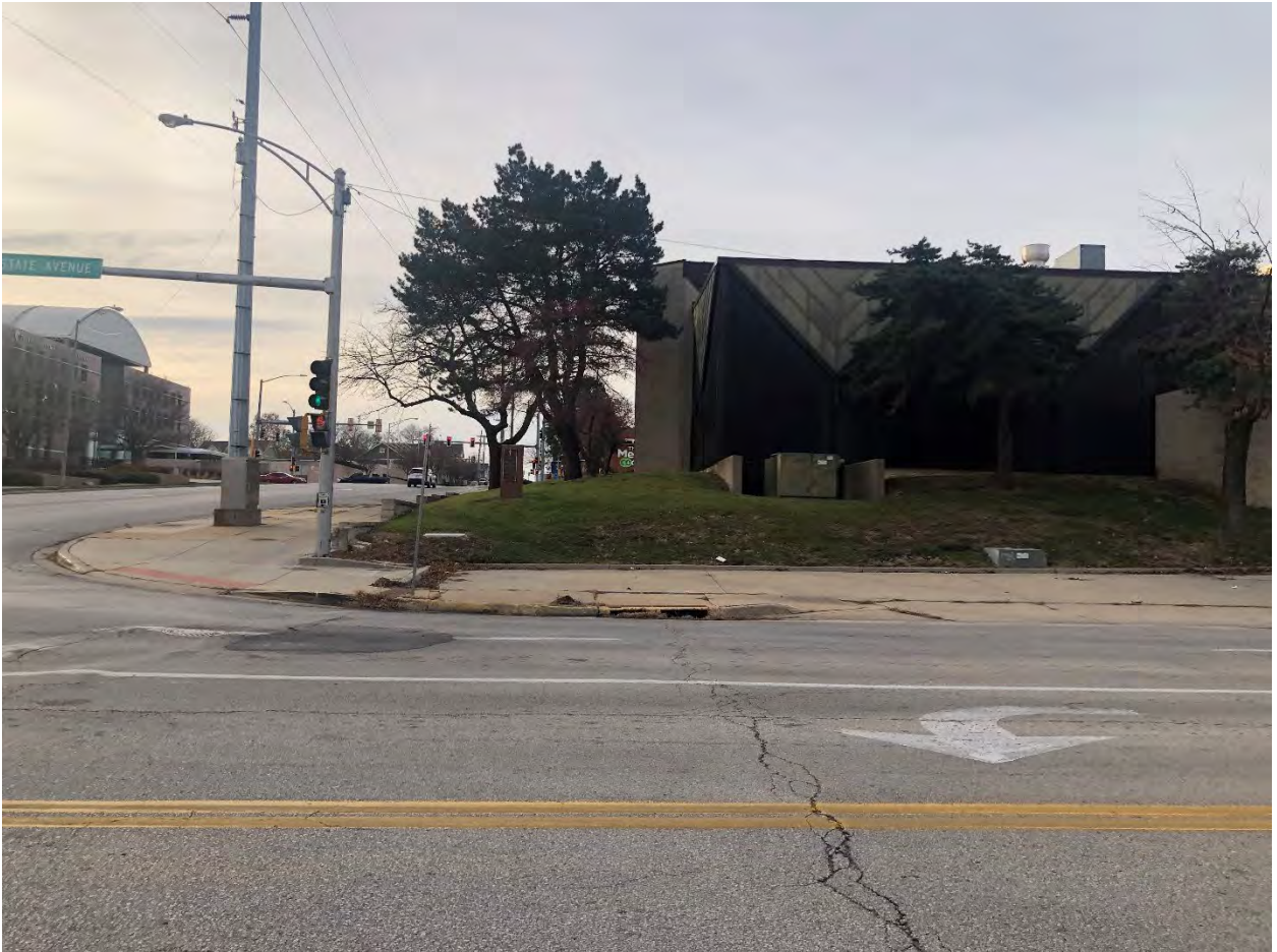
Figure 6. Site Photograph of the Reardon Civic Center from State Avenue looking south (provided by Planning Staff).
