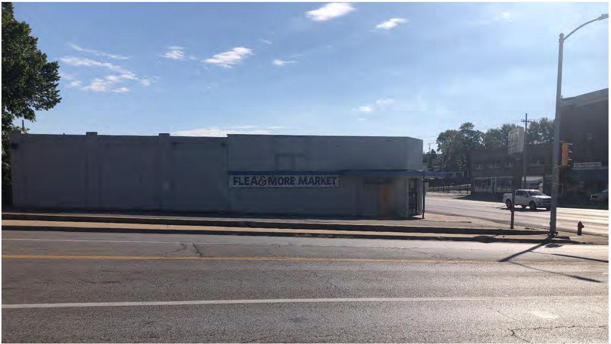
Figure 6. Site photograph of 1720 Minnesota Avenue looking east taken from North 18 th Street (provided by Planning Staff).
