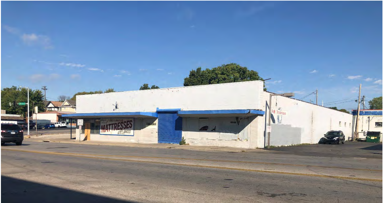
Figure 4. Site photograph of 1720 Minnesota Avenue looking northwest taken from Minnesota Avenue (provided by Planning Staff).
