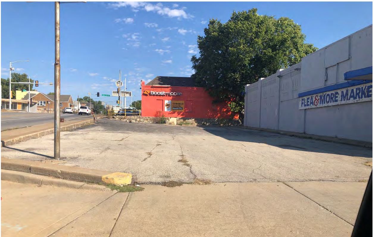
Figure 5. Site photograph of 1720 Minnesota Avenue looking north taken from Minnesota Avenue (provided by Planning Staff).
