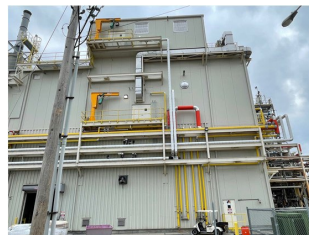
After with building enclosed.
