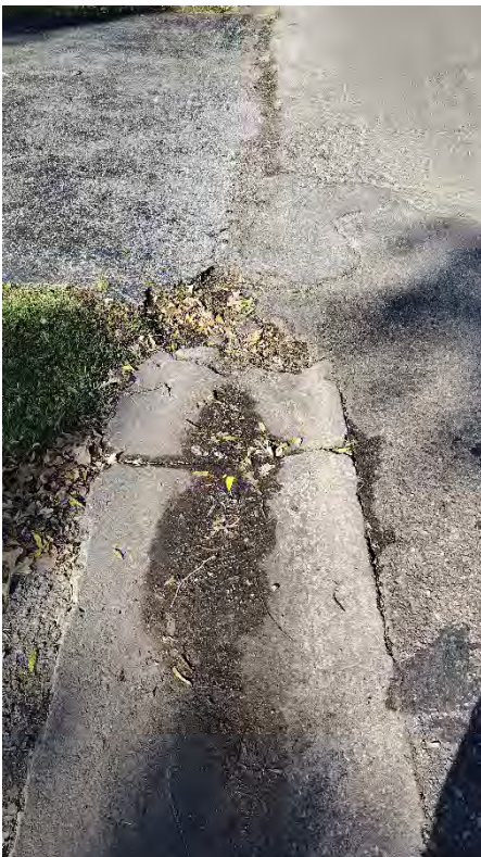
Left: The subject driveway was paved with asphalt improperly, and in doing so has covered the curb-gutter stormwater system that serves Shawnee Road. Applicant stated that neither they nor the property owner paved the driveway—rather, that it had been paved by the previous property owner—but that they are willing to repair the curb, as the backed-up surface water has had a negative effect on the subject property's front lawn.
