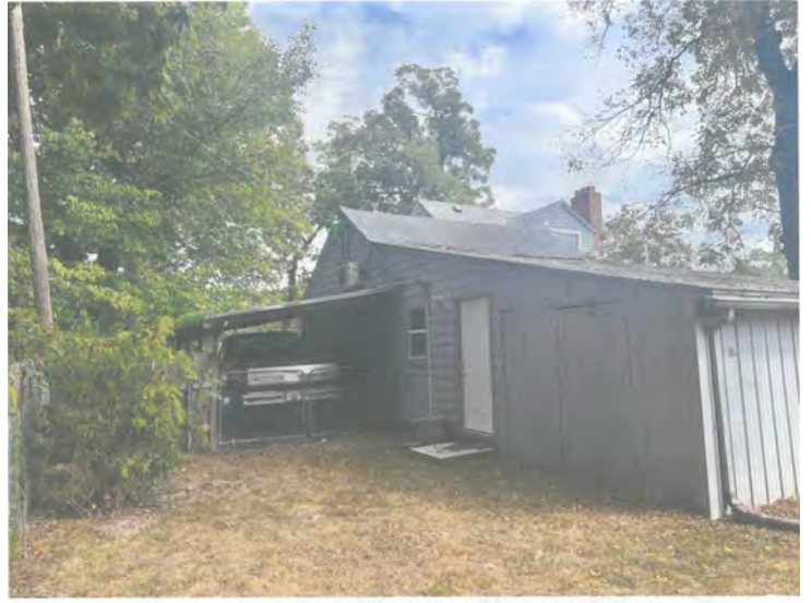
North Side of House with Door to Workshop
