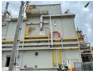
After with building enclosed.
