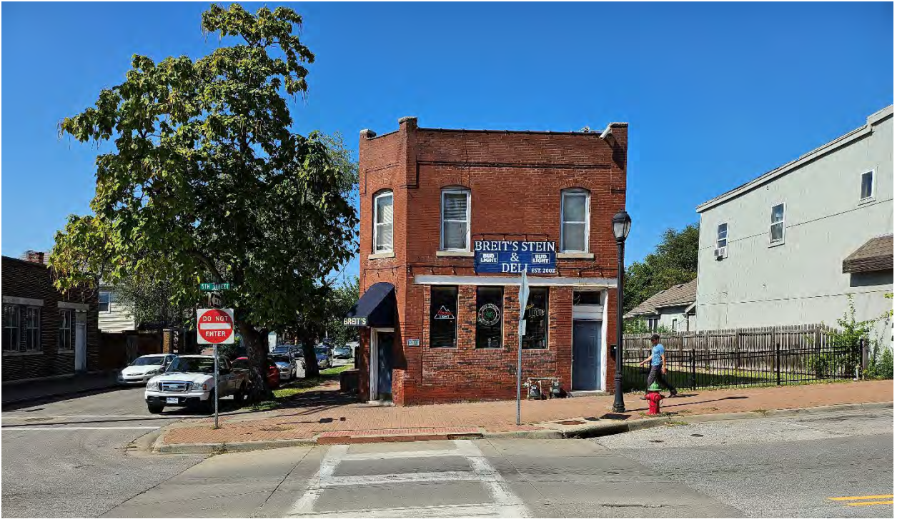
Figure 4. Site Photograph of 412 North 5 th Street looking west from North 5 th Street (provided by the Applicant).
