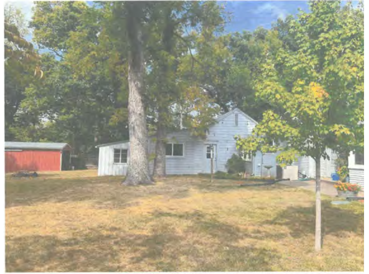
South Side of House with Door to Garage
