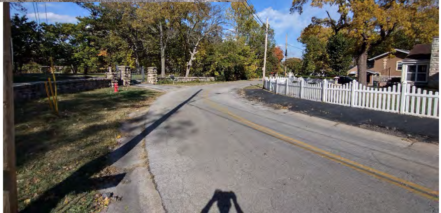
Left: The subject driveway was paved with asphalt improperly, and in doing so has covered the curb-gutter stormwater system that serves Shawnee Road. Applicant stated that neither they nor the property owner paved the driveway—rather, that it had been paved by the previous property owner—but that they are willing to repair the curb, as the backed-up surface water has had a negative effect on the subject property's front lawn.
