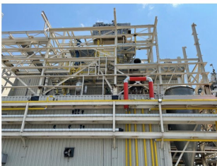
Before with initial steel and some major equipment set.
