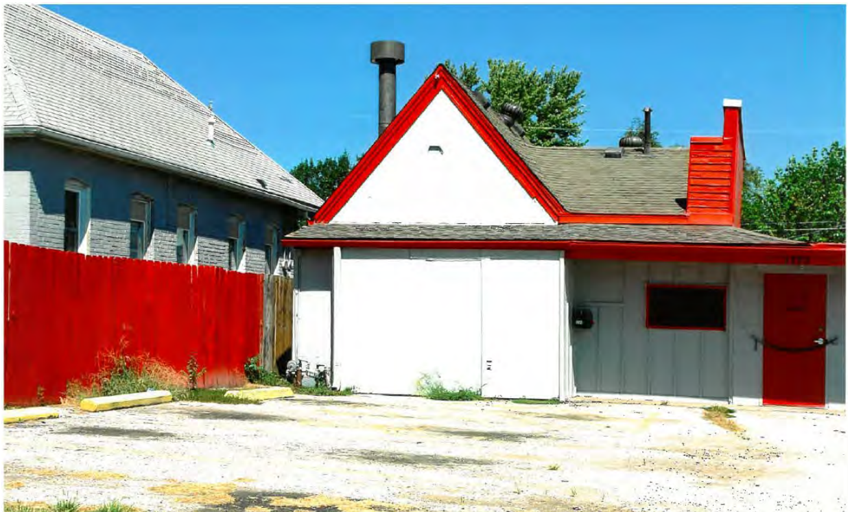
Figure 5. Site Photograph of 1200 Osage Avenue looking north from Osage Avenue (provided by the Applicant).
