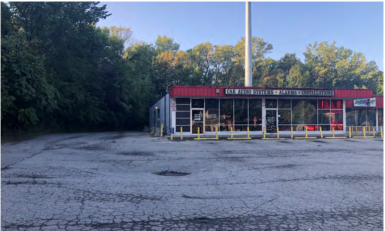
Figure 5. Site Photograph of 5235 State Avenue looking south from State Avenue (provided by Planning Staff).
