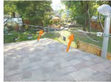
3 Feet Clearance Recommended
