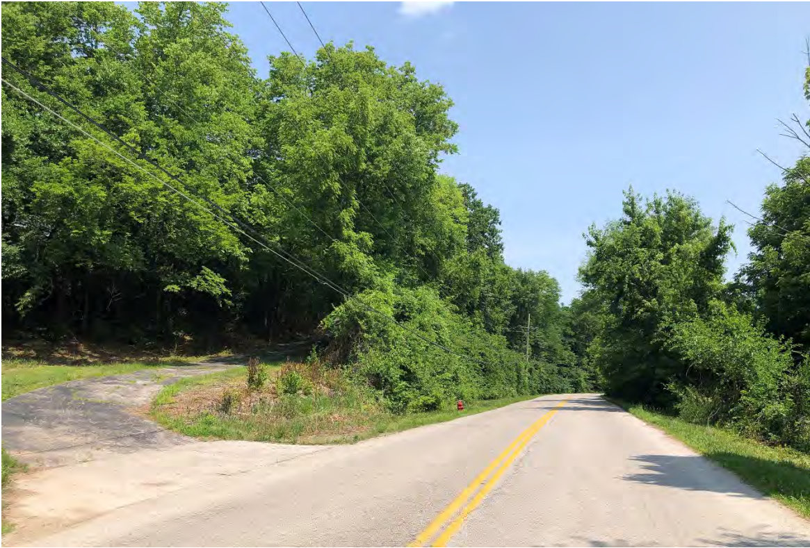
Figure 6. Site photograph looking north on North 55 th Street (provided by Planning Staff).
