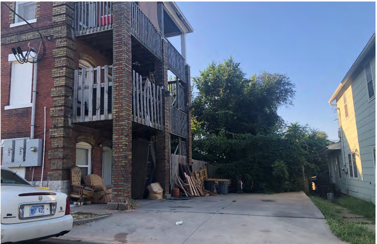
Figure 5. Site Photograph of 612 North 5th Street looking south from Barnett Avenue (provided by Planning Staff).
