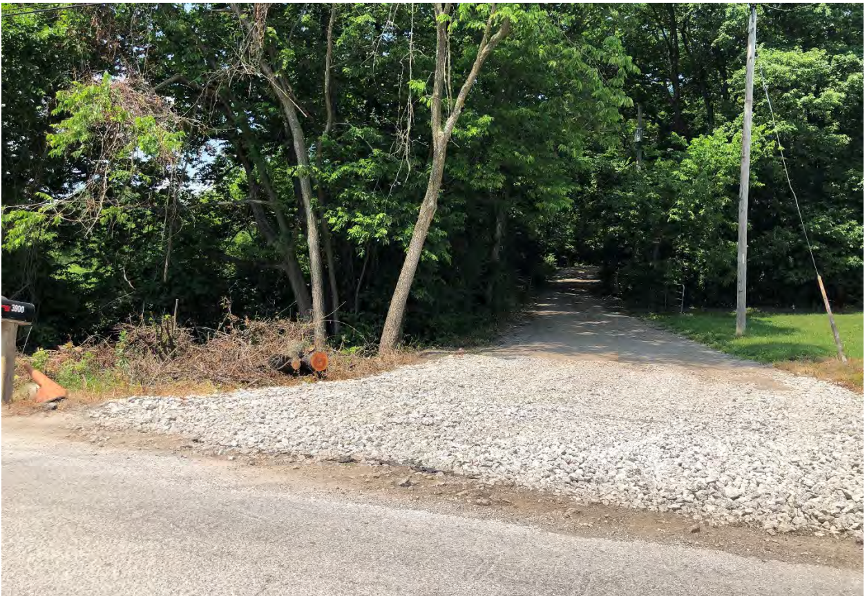
Figure 5. Site photograph looking west at 3850 North 55th Street (provided by Planning Staff).
