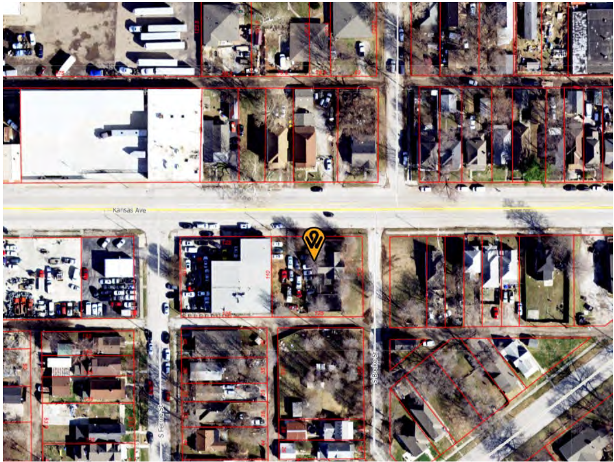
Figure 1. Aerial photograph of 927 Kansas Avenue (provided by UG Maps).
