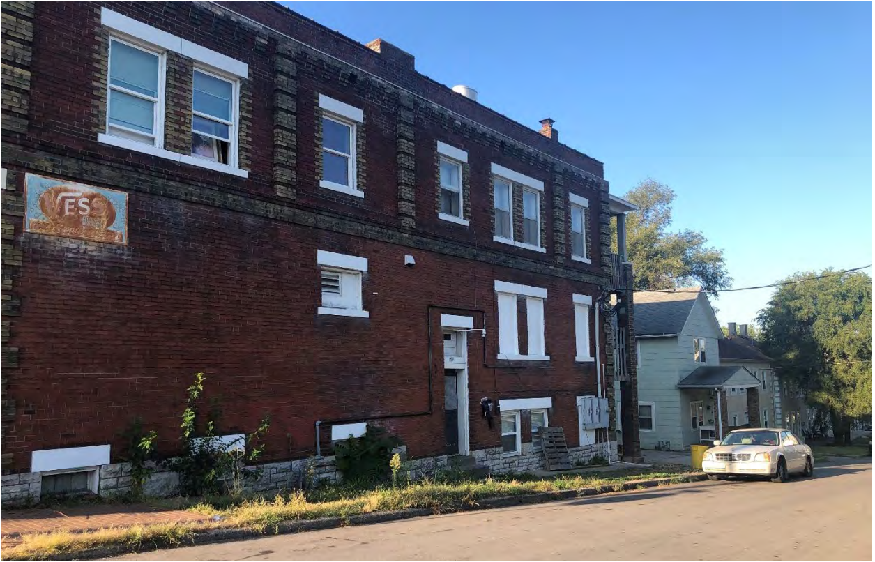
Figure 6. Site Photograph of 612 North 5th Street looking southwest from Barnett Avenue (provided by Planning Staff).
