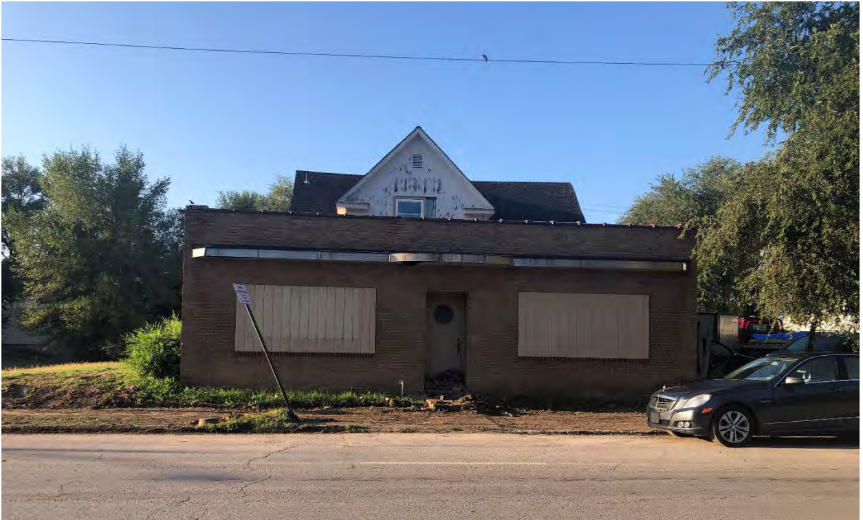
Figure 5. Site Photograph of 927 Kansas Avenue looking south from Kansas Avenue (provided by Planning Staff).
