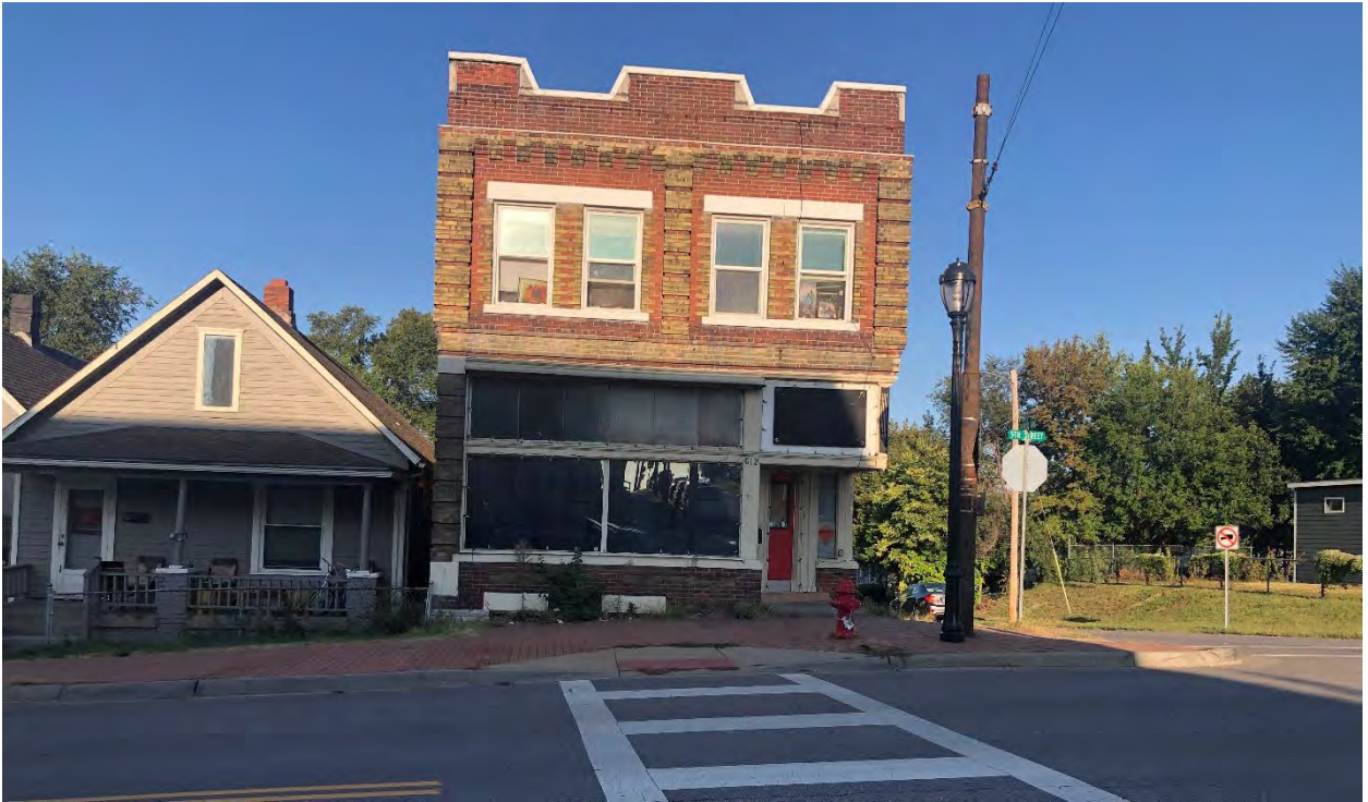
Figure 4. Site Photograph of 612 North 5 th Street looking west from North 5 th Street (provided by Planning Staff).
