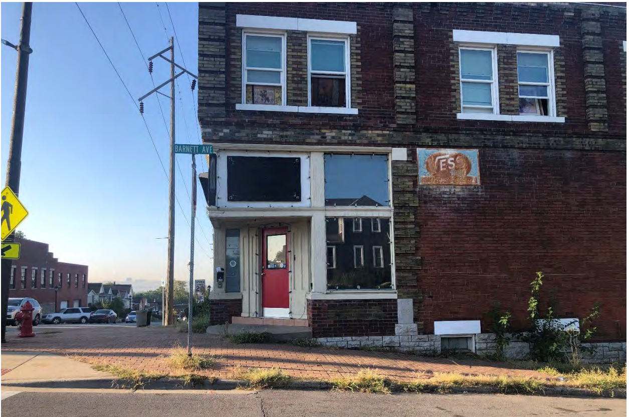
Figure 5. Site Photograph of 612 North 5 th Street looking south from Barnett Avenue (provided by Planning Staff).
