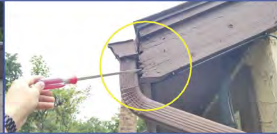
Rear NE corner
