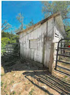
Current shed on Parcel 922535
