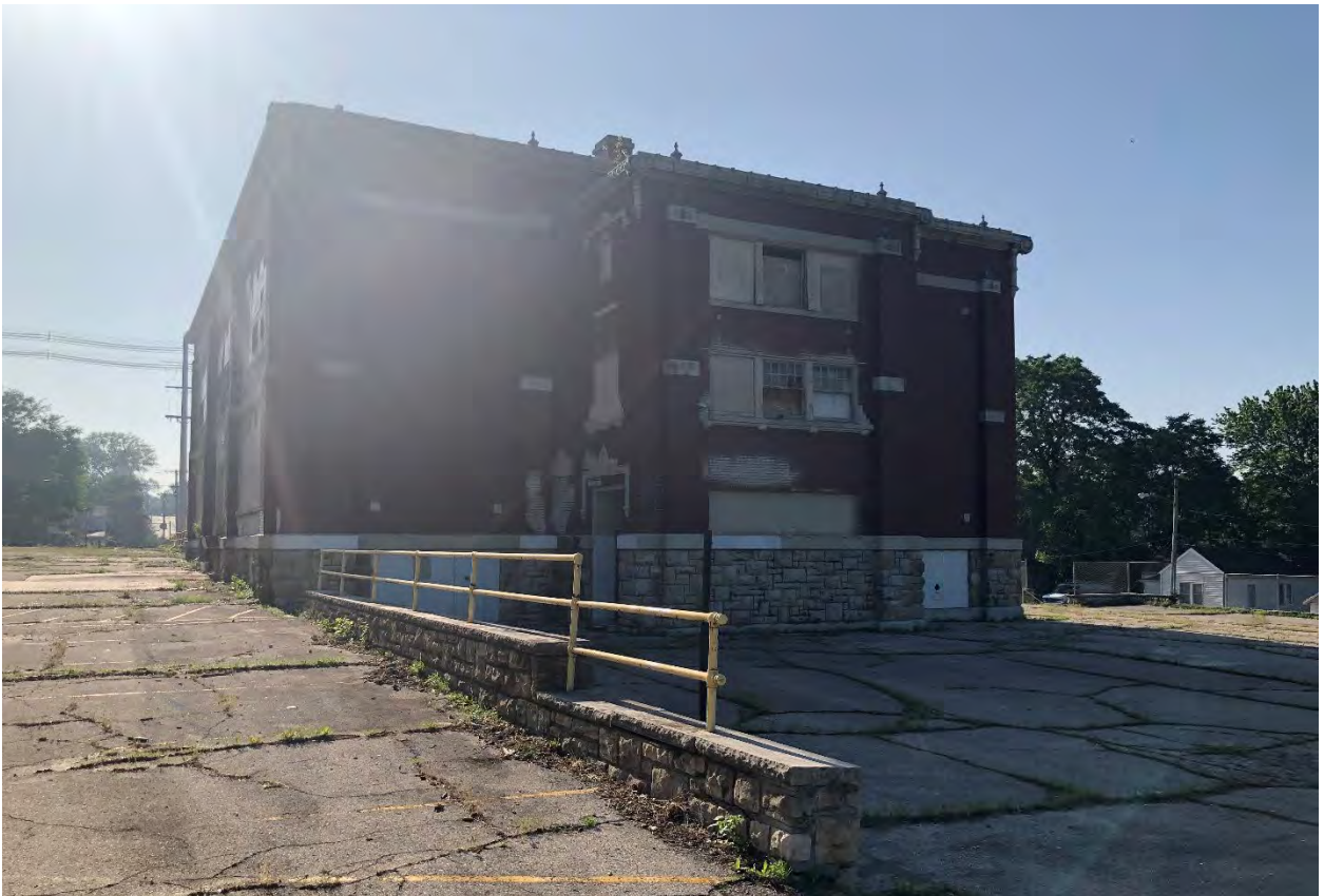
Figure 7. Site Photograph of 290 South 10th Street looking southeast (provided by Planning Staff).
