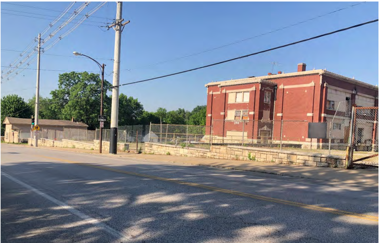
Figure 9. Site Photograph of 290 South 10th Street looking southwest (provided by Planning Staff).
