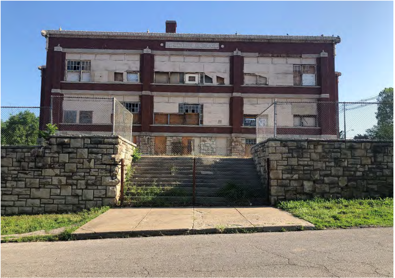
Figure 4. Site photograph looking north at 290 South 10 th Street (provided by Planning Staff).
