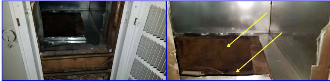
Exposed wood and floor for intake
