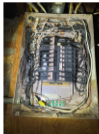
Manufacturer and Size: Cutler Hammer - 100 amps
