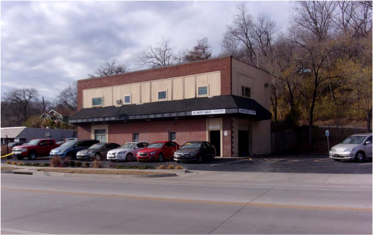
Figure 4. Site Photograph of 1010 Merriam Lane taken on November 20, 2020.
