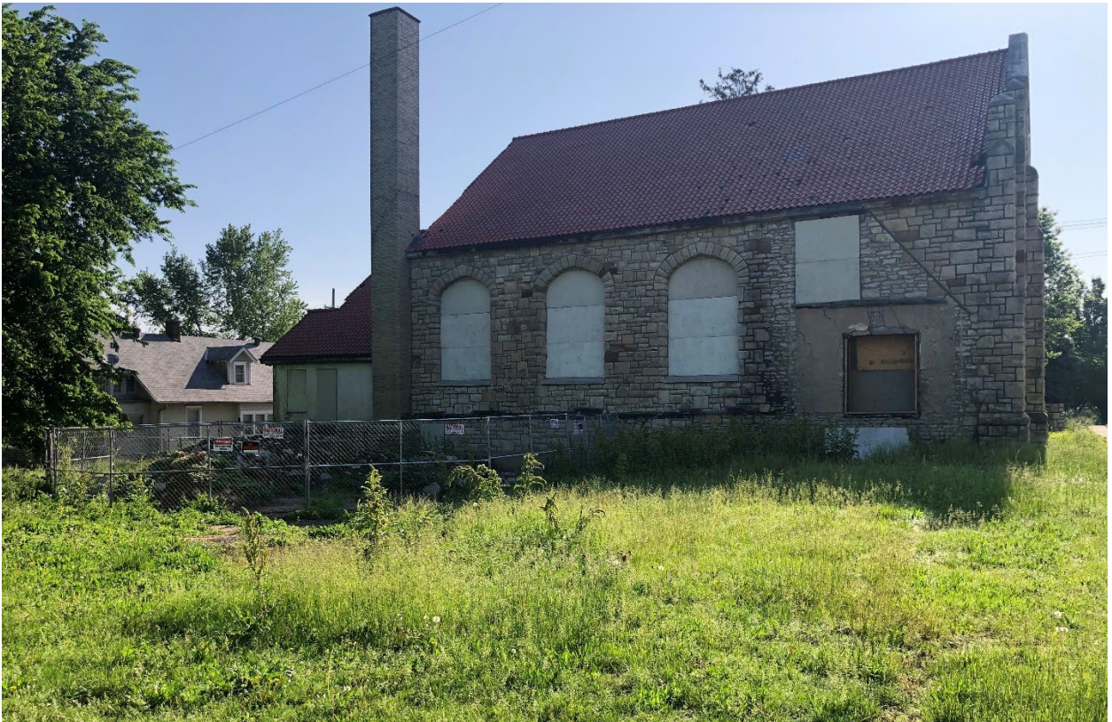
Figure 5. Site photograph of 2508 North 10 th Street and 1208 Cleveland Avenue looking east (provided by Planning Staff).
