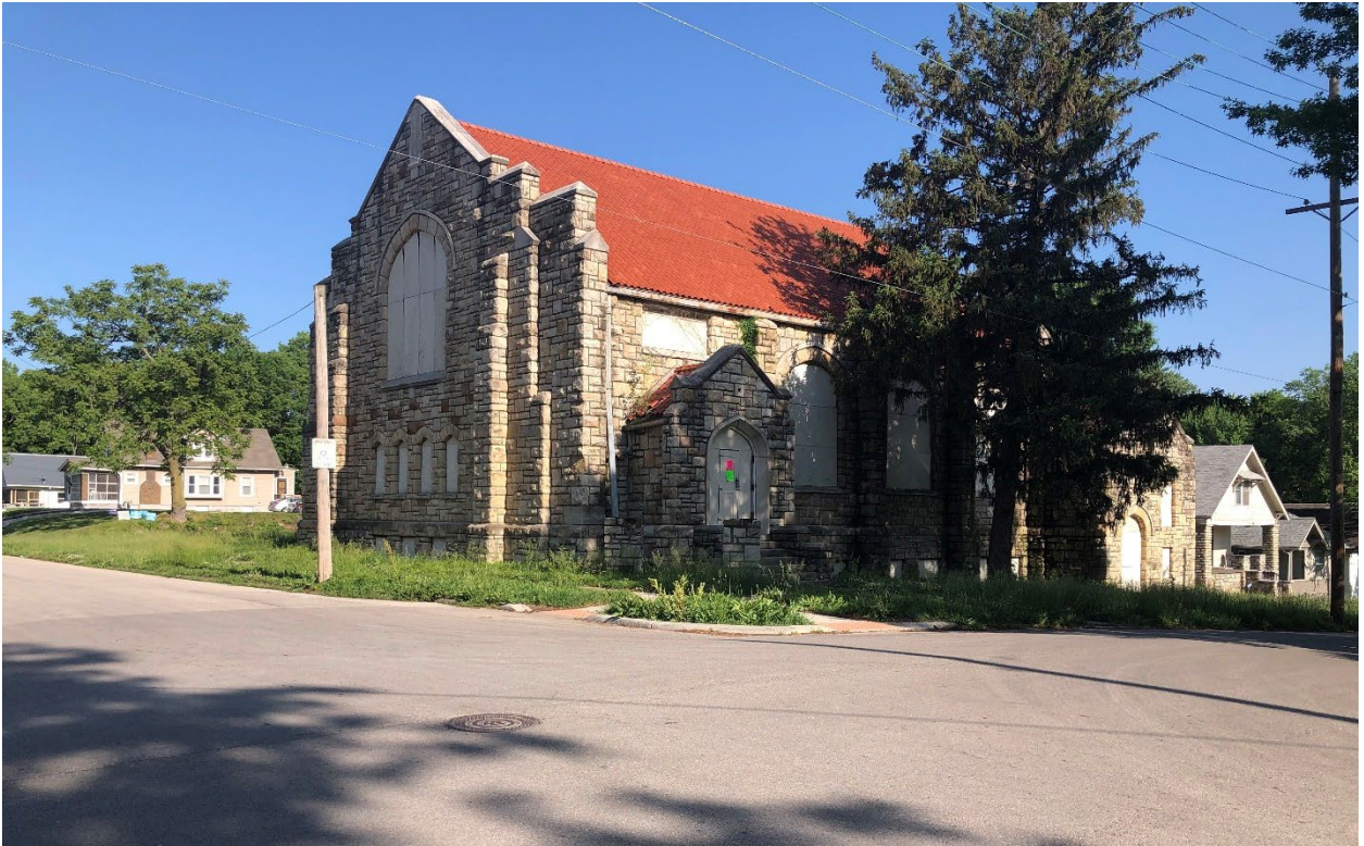
Figure 4. Site photograph of 2508 North 10 th Street and 1208 Cleveland Avenue looking northwest (provided by Planning Staff).
