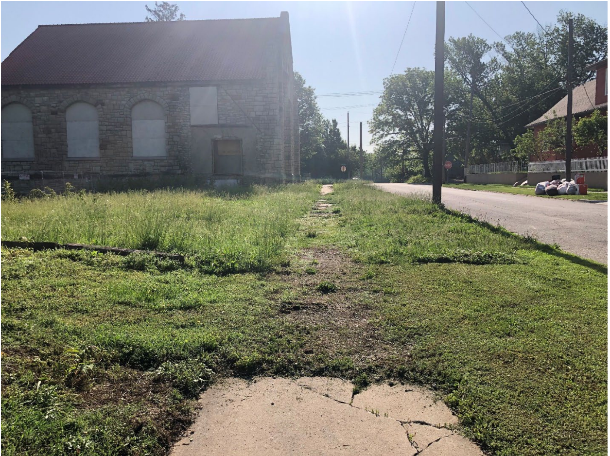
Figure 6. Site photograph of 2508 North 10 th Street and 1208 Cleveland Avenue looking east (provided by Planning Staff).
