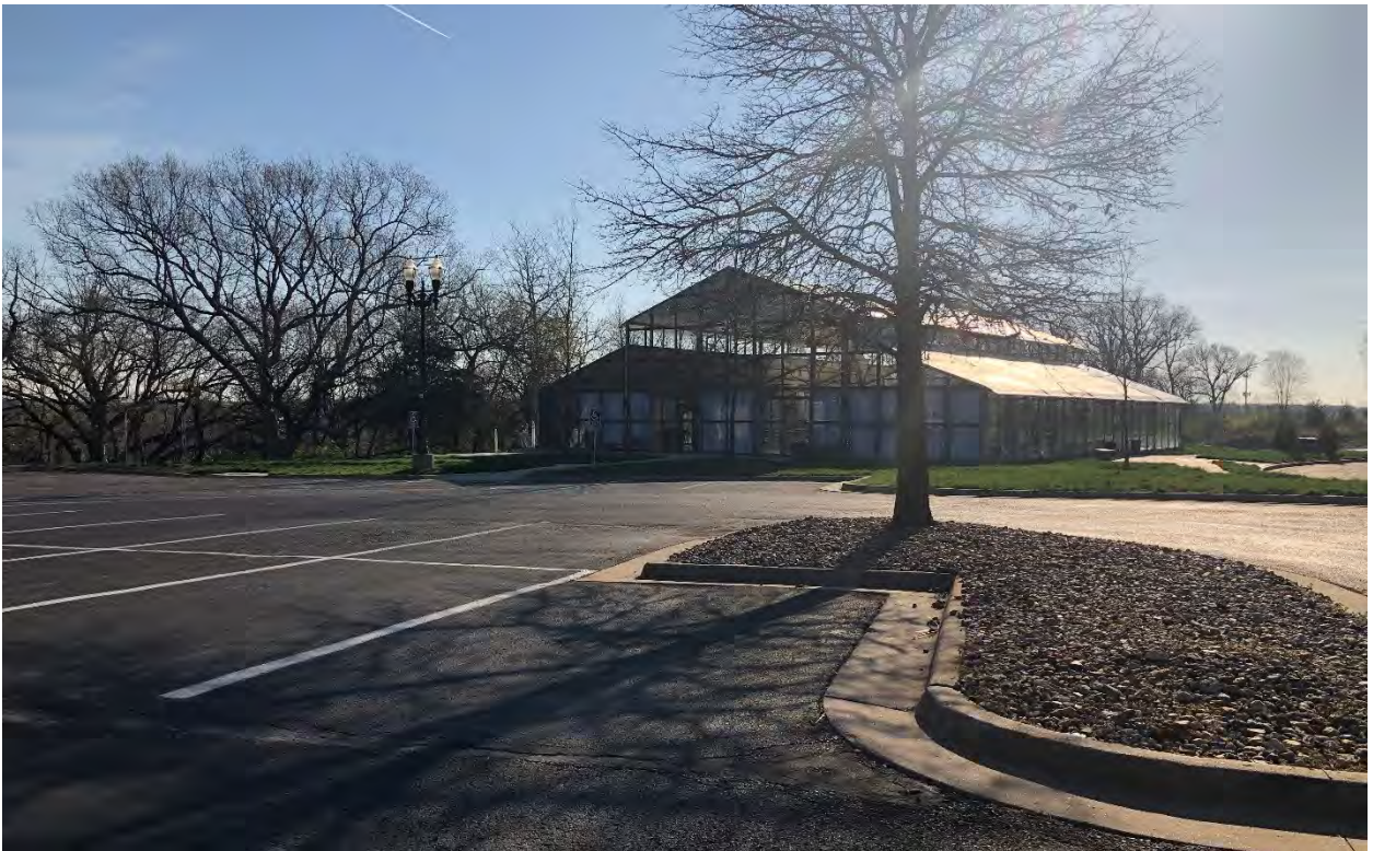
Figure 5. Site Photograph of 701 Village West Parkway looking northeast (provided by Planning Staff).
