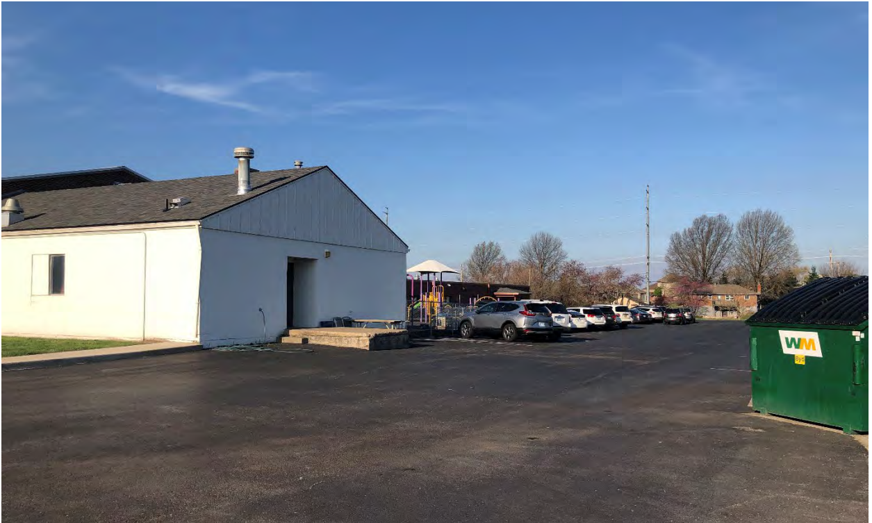
Figure 6. Site Photograph of 3130 North 122nd Street looking southwest (provided by Planning Staff).
