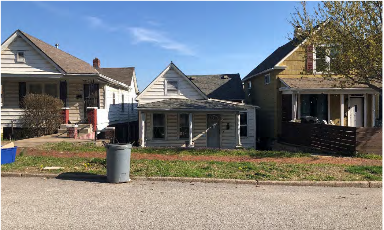
Figure 5. Site Photograph of 410 Ann Avenue looking north from Ann Avenue (provided by Planning Staff).
