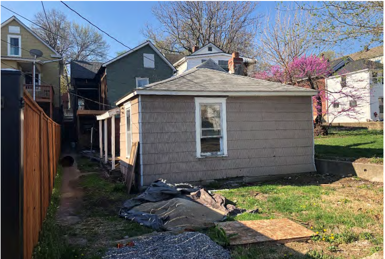
Figure 6. Site Photograph of 410 Ann Avenue looking south taken from the alley (provided by Planning Staff).
