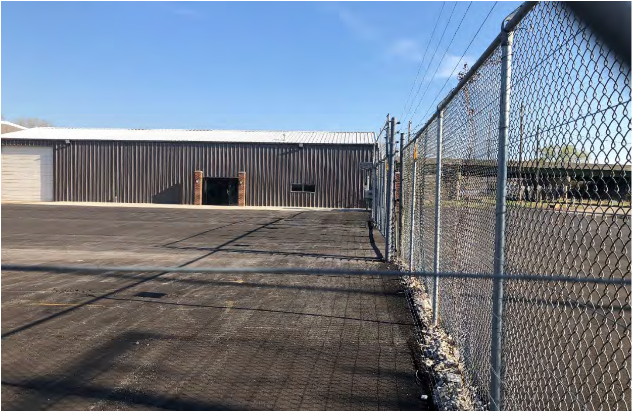
Figure 7. Site Photograph of 336 South 42nd Street looking north (provided by Planning Staff).
