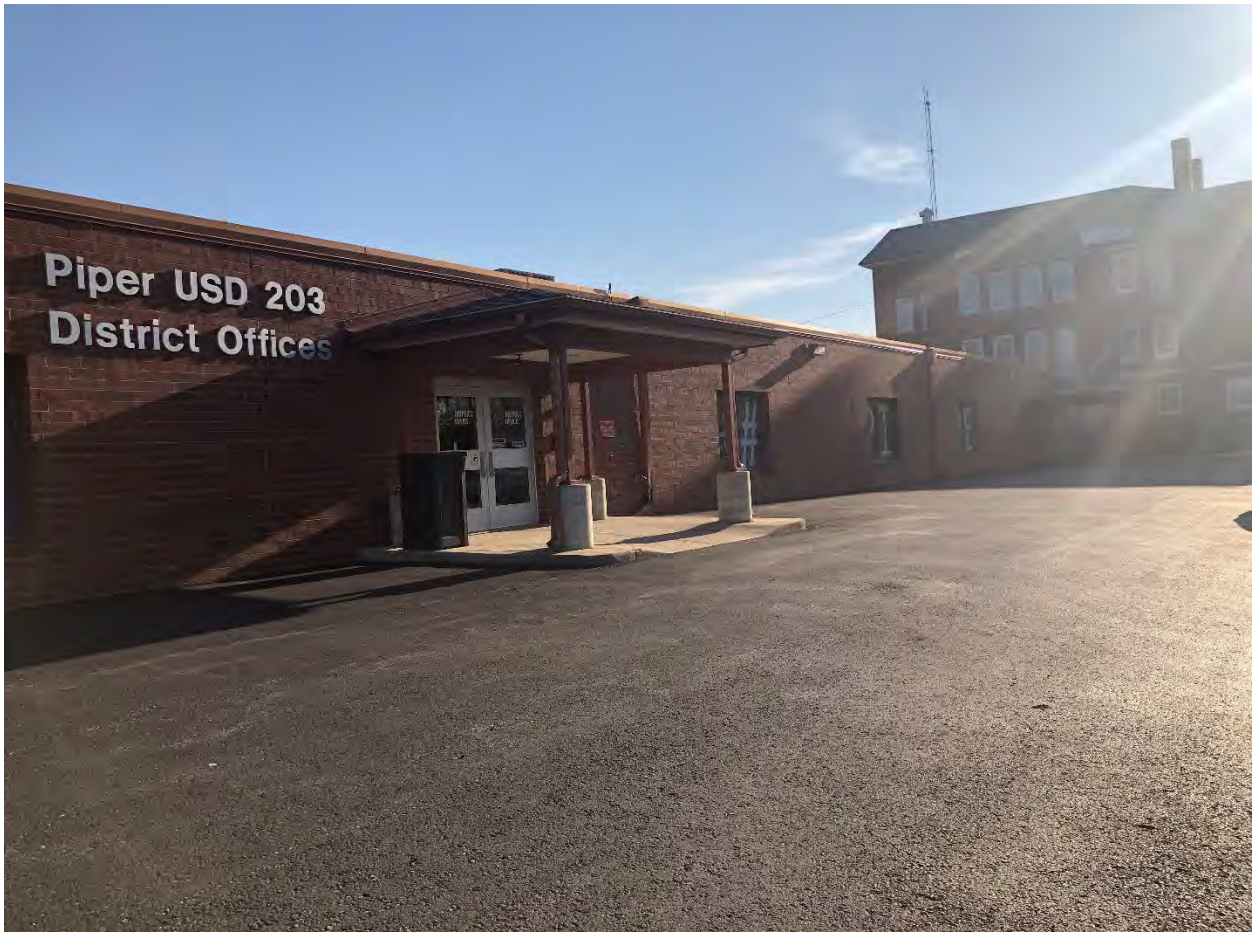
Figure 4. Site Photograph of 3130 North 122nd Street looking east (provided by Planning Staff).
