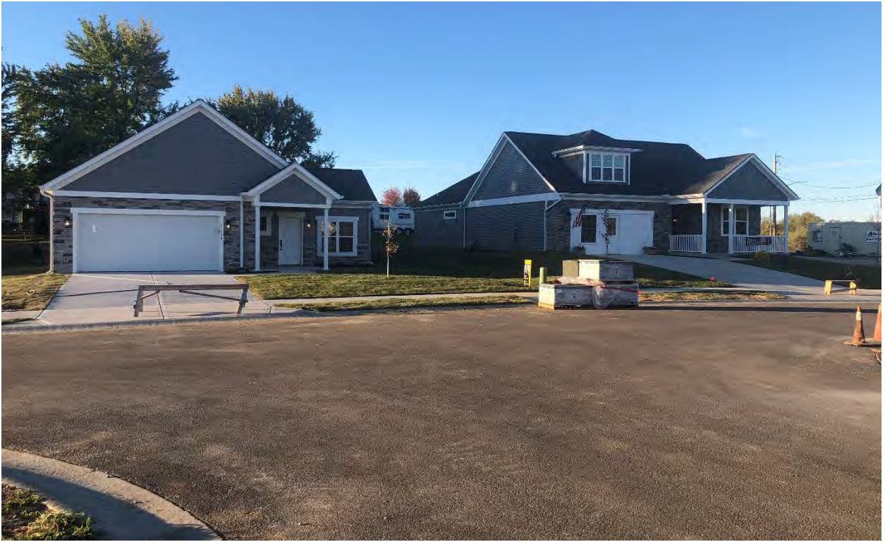
Figure 4. Site Photograph of Villas of Piper Valley, Phase 1 looking south (provided by Planning Staff).
