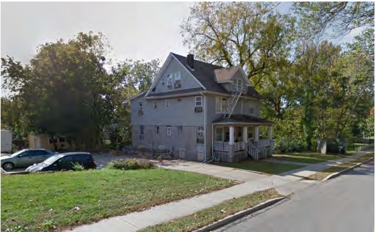
Figure 5. Site photograph looking southwest at 915 Barnett Avenue (provided by Planning Staff).
