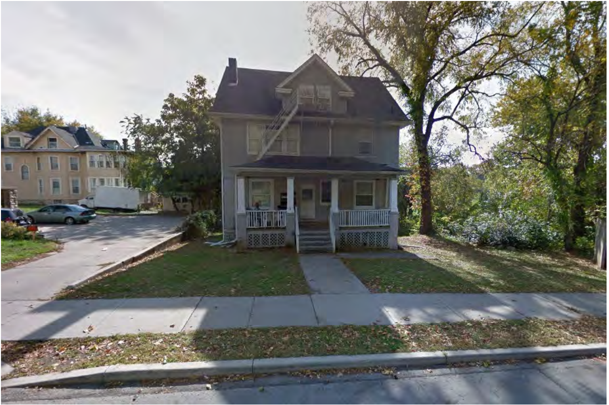
Figure 4. Site photograph looking south at 915 Barnett Avenue (provided by Planning Staff).
