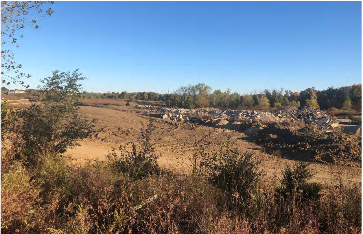
Figure 5. Site photograph of 9400 State Avenue looking north (provided by Planning Staff).
