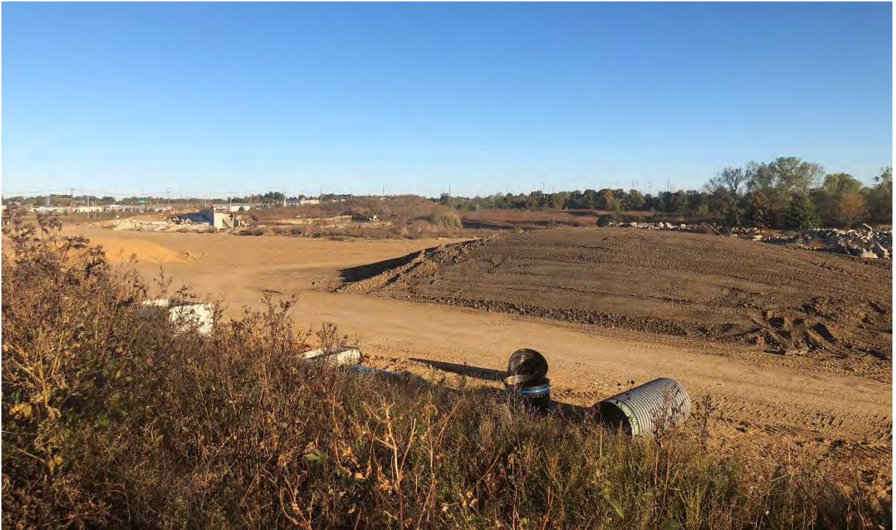
Figure 4. Site photograph of 9400 State Avenue looking northwest (provided by Planning Staff).
