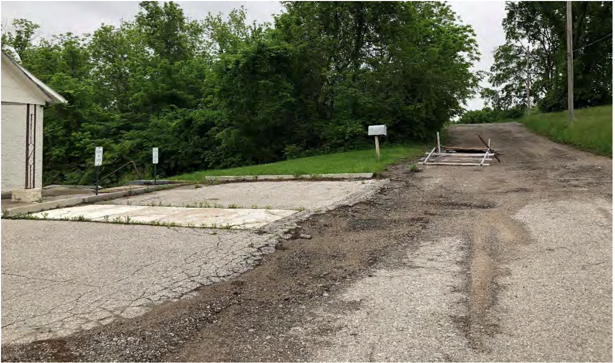
Figure 4. Site Photograph of North 49th Terrace looking south (provided by Staff).
