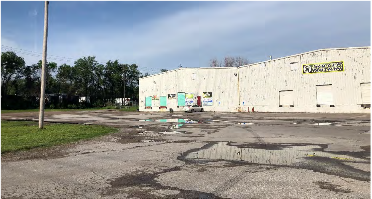
Figure 4. Site photograph looking northwest at 520 South 55 th Street taken on May 18, 2022.
