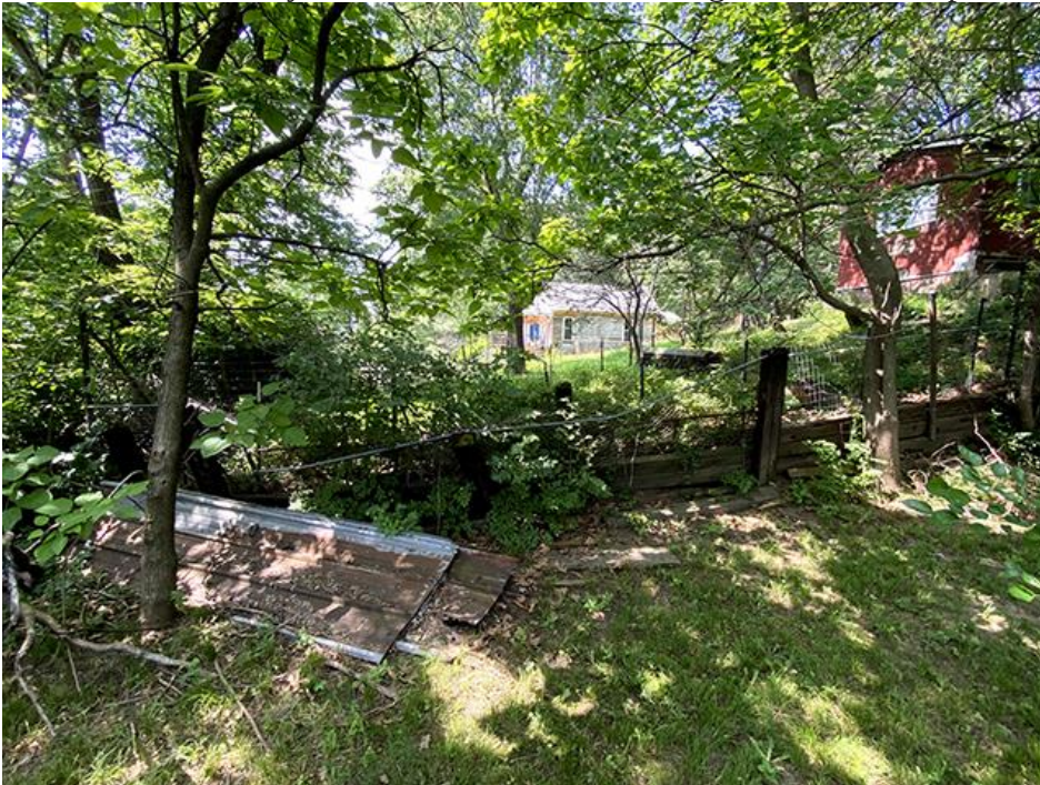
Photo 06: Deteriorated or deteriorating structures, unsanitary or unsafe conditions
