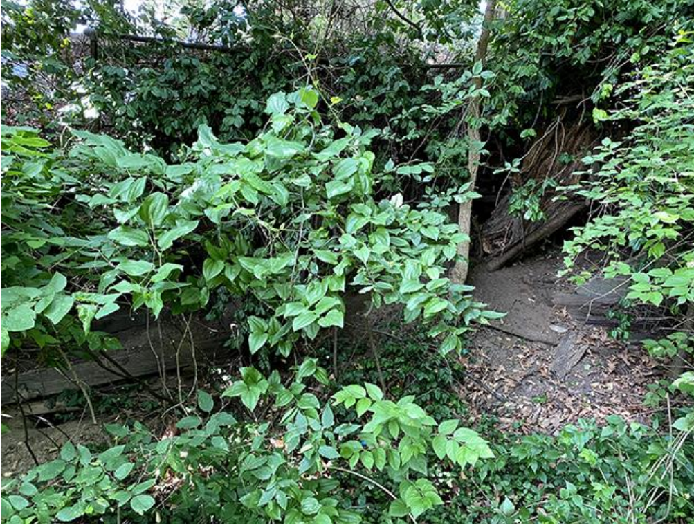
Photo 09: Deteriorated or deteriorating structures, unsanitary or unsafe conditions
