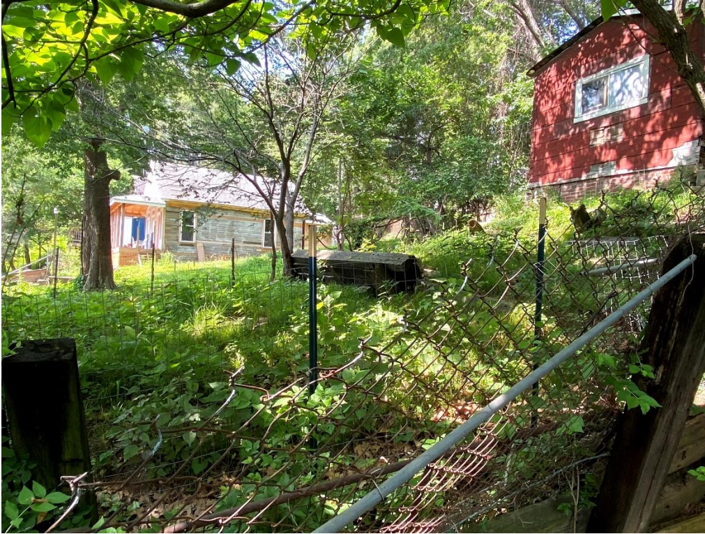
Photo 07: Deteriorated or deteriorating structures, unsanitary or unsafe conditions
