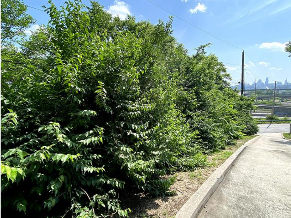
Photo 05: Unsanitary or unsafe conditions – Overgrown trees into power lines
