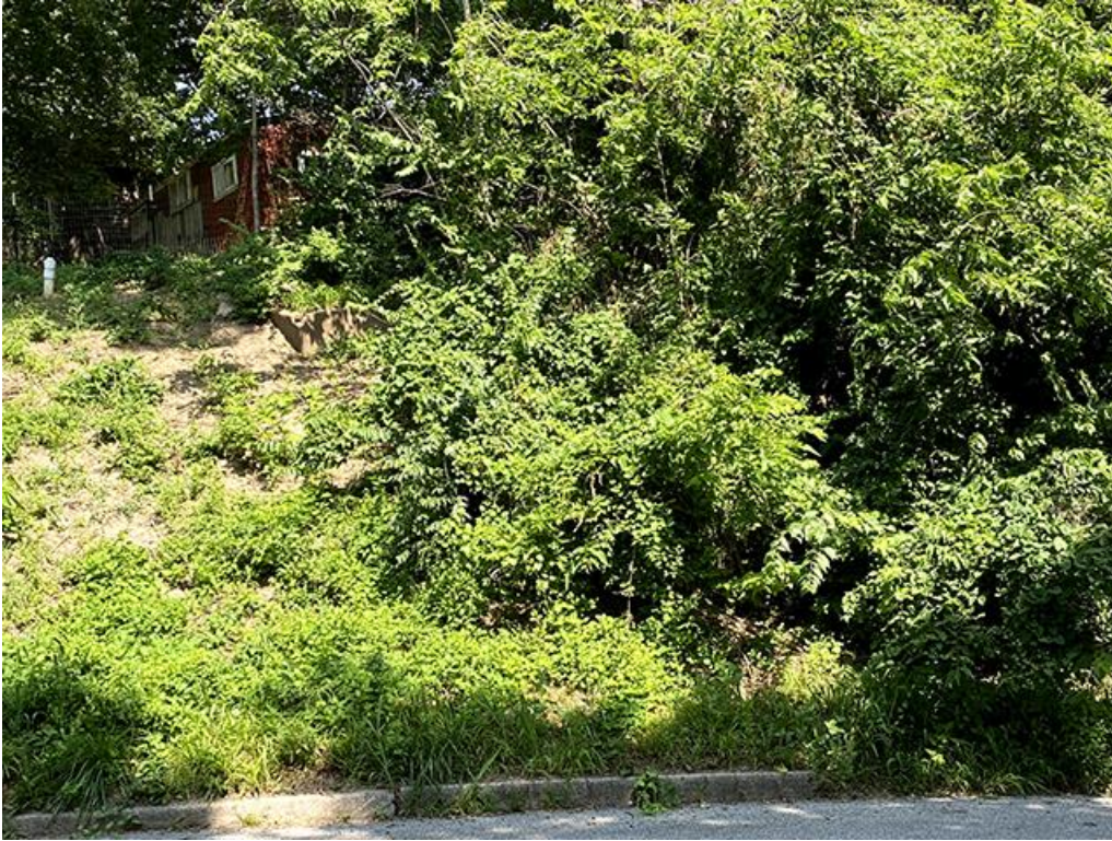
Photo 03: Deterioration of site improvements - No sidewalks, overgrown weeds, erosion
