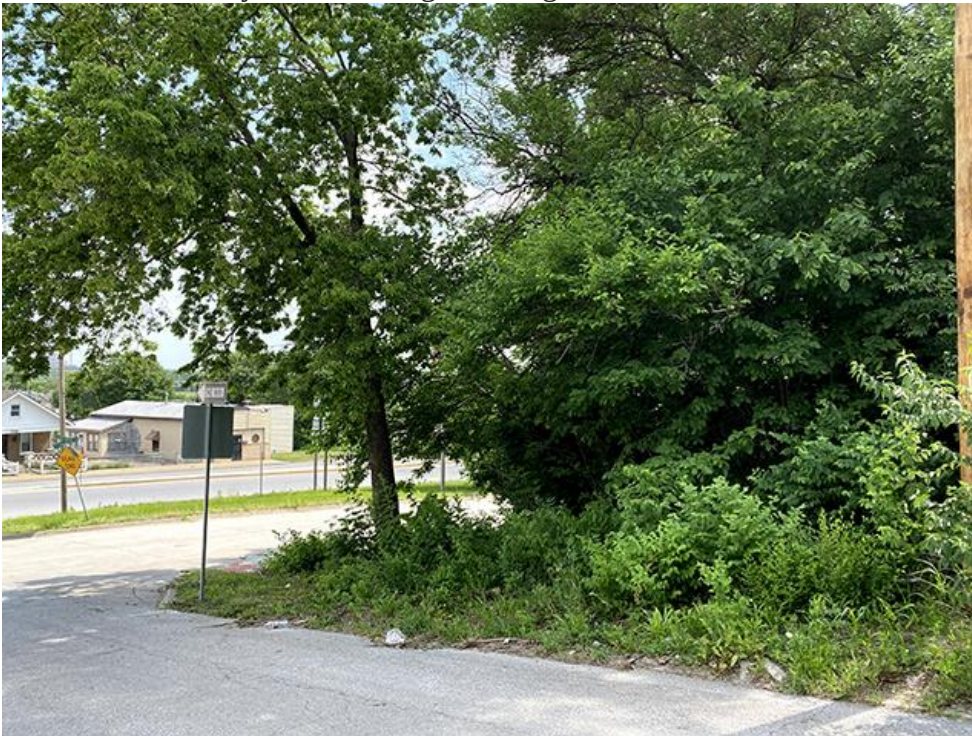
Photo 12: Deterioration of site improvements - No sidewalks, overgrown weeds, erosion
