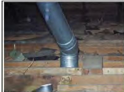
Flue pipe in attic
