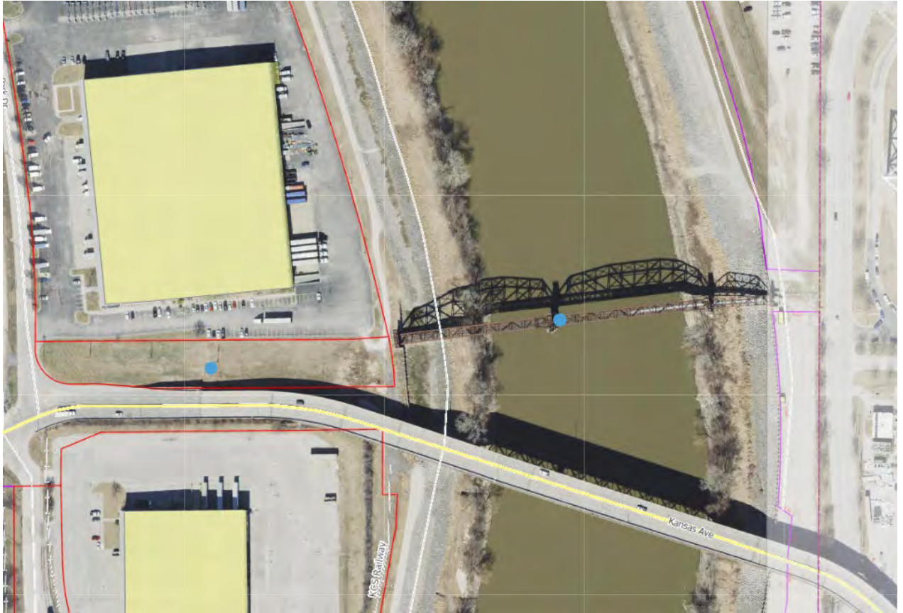
Figure 1. Aerial Photograph of 557 River Park Drive and 0 Kansas Avenue (proposed address for Rock Island Bridge) as indicated by the blue dots (provided by UG Maps).
