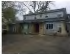
2100 Washington Blvd. South elevation. 4/2019. Tax Credit Application.
