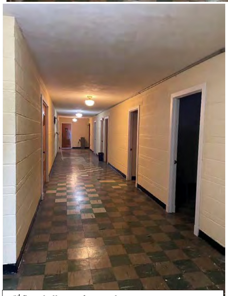
2 nd floor hallway of more classrooms.
