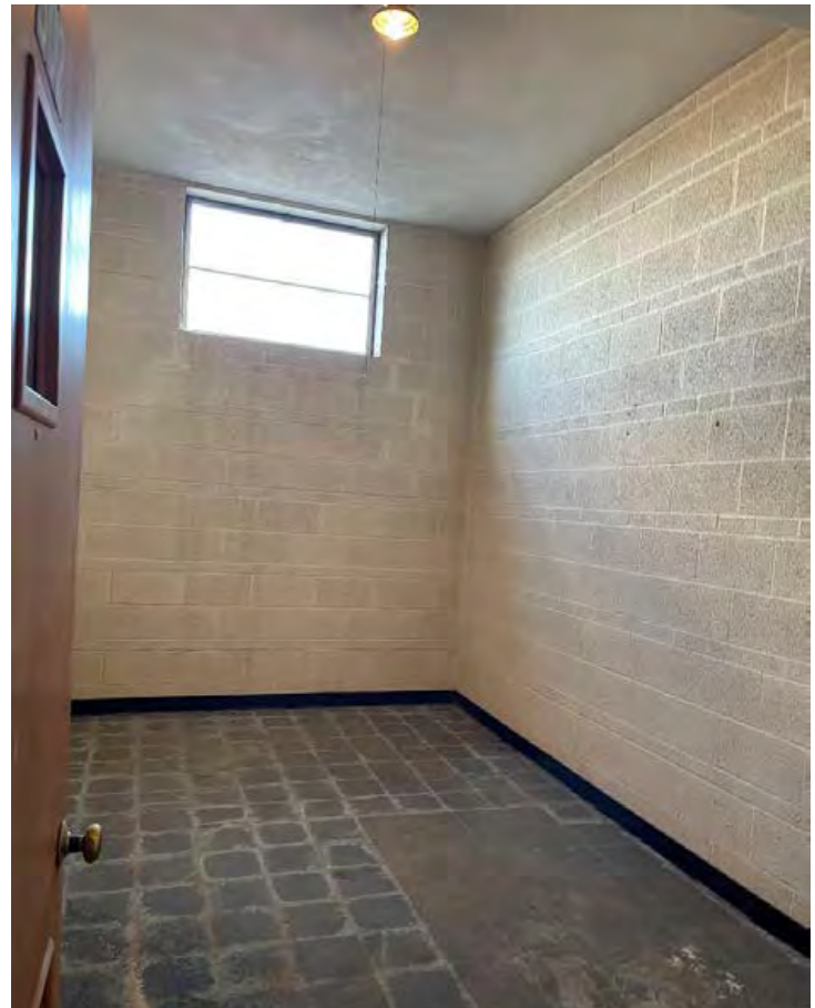
Example of 3 rd floor classroom.
