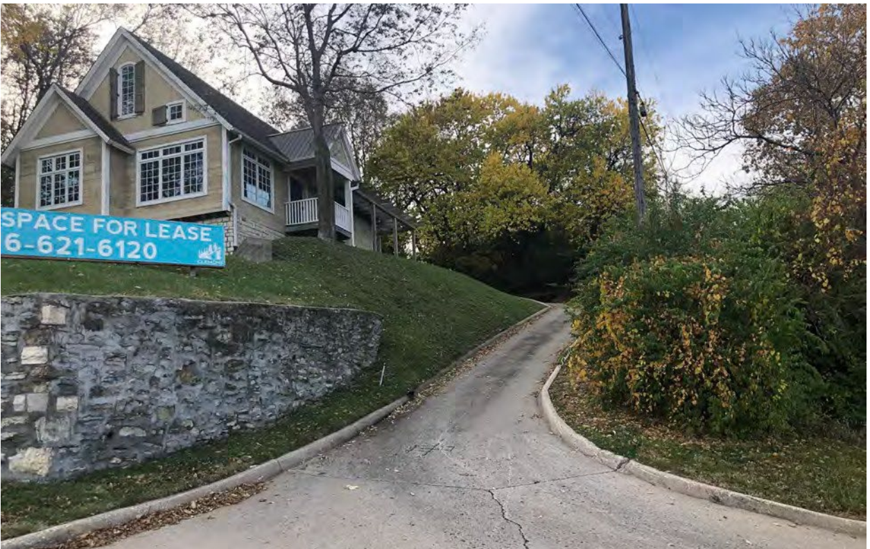
Figure 9. Site Photograph of 10 South Hallock Street looking west (provided by Planning Staff).
