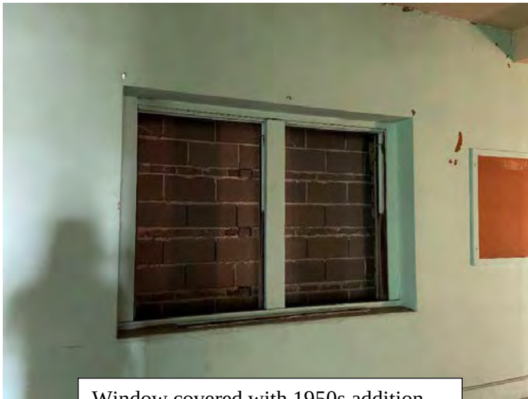
Window covered with 1950s addition.
