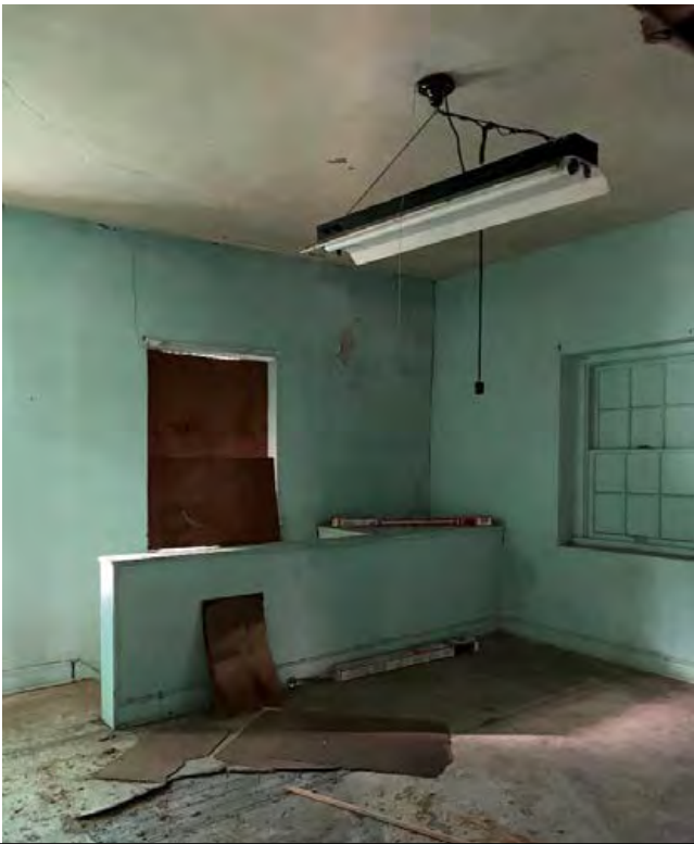
3 rd floor classroom space.
