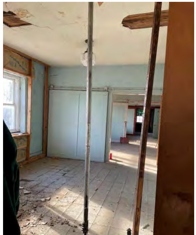
3 rd floor classrooms on old side of building. Note rolling door divisions.
