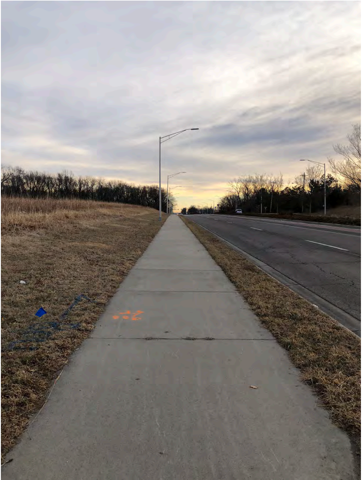
Figure 5. Site photograph looking east on State Avenue at 9020 State Avenue taken on January 12, 2022.
