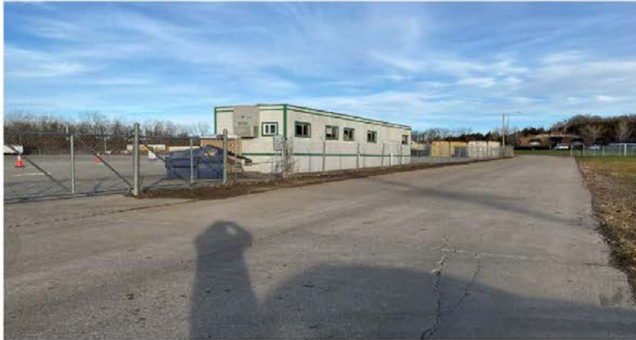
Entry to Site looking North
