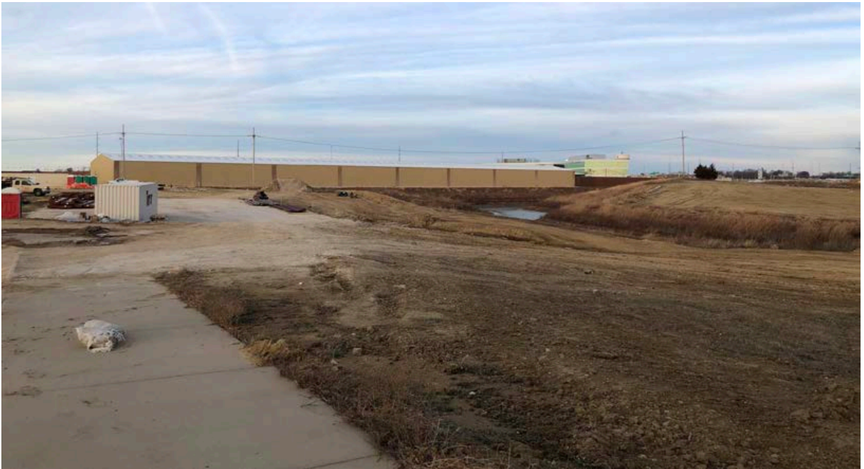
Figure 2. Site photograph looking west at 9400 State Avenue.
