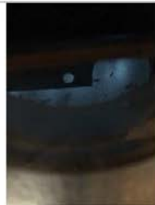
Furnace fired correctly at time of inspection.
