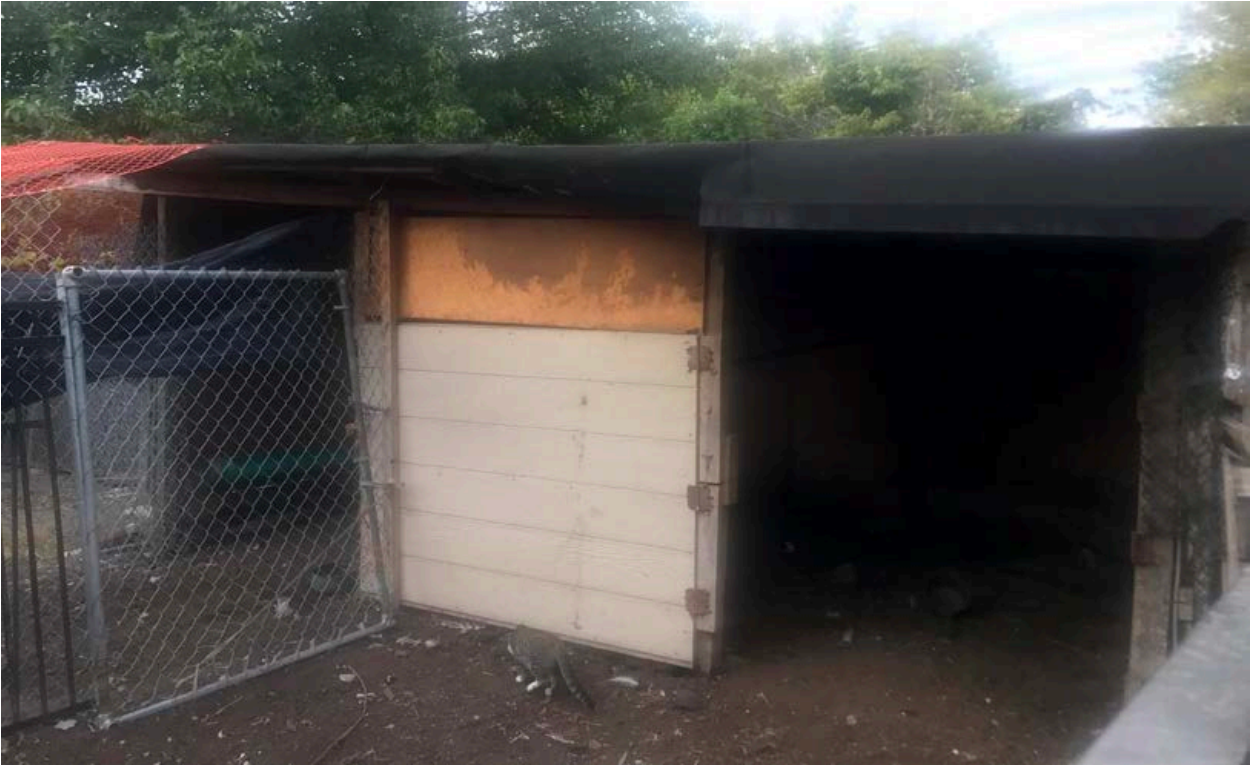
Figure 6. Photograph of an accessory structure at 3740 North 35th Street (provided by the applicant).
