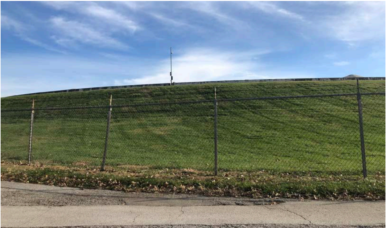
Figure 9. Site Photograph of 1801 South 14th Street looking east from Lawrence Avenue (provided by Staff).
