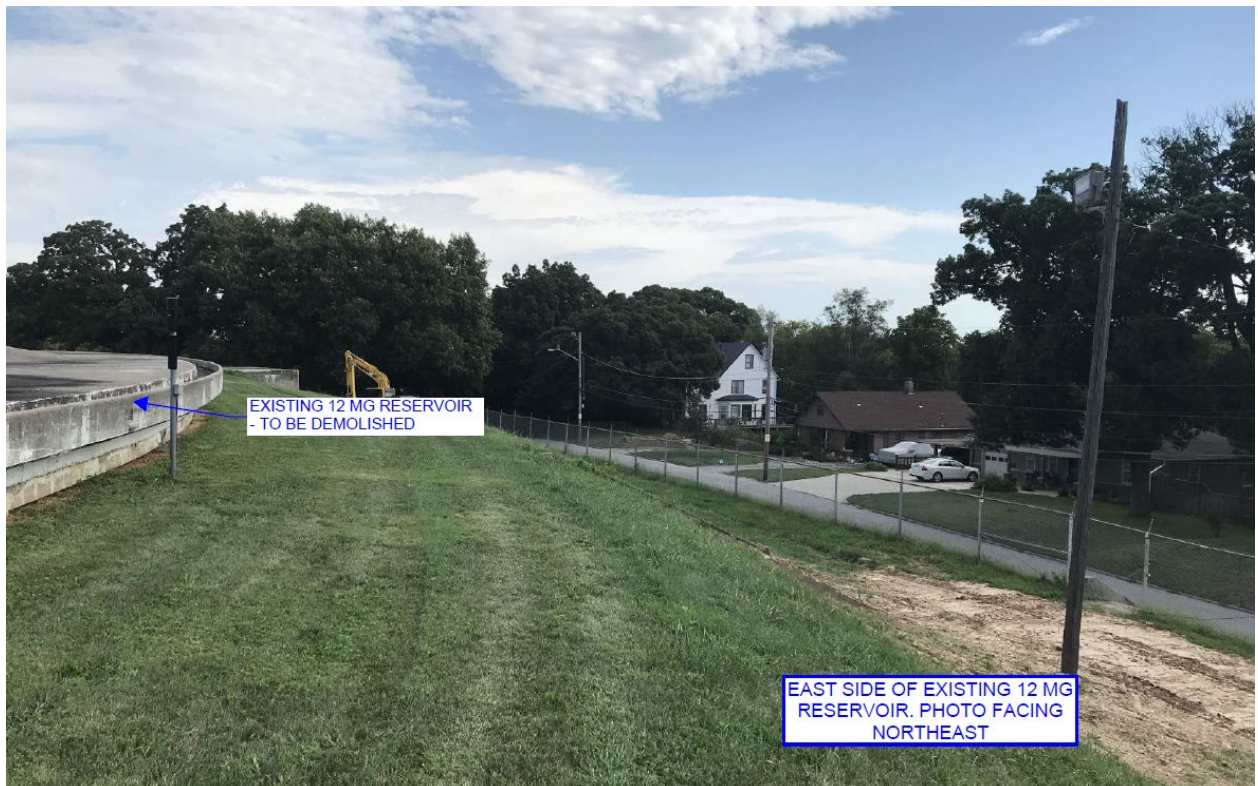
Figure 6. Photograph of 1801 South 14th Street (provided by the applicant).
