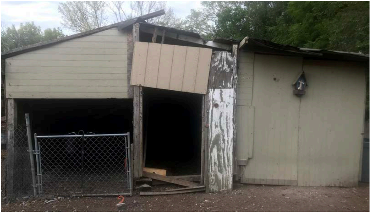
Figure 4. Photograph of an accessory structure at 3740 North 35th Street (provided by the applicant).
