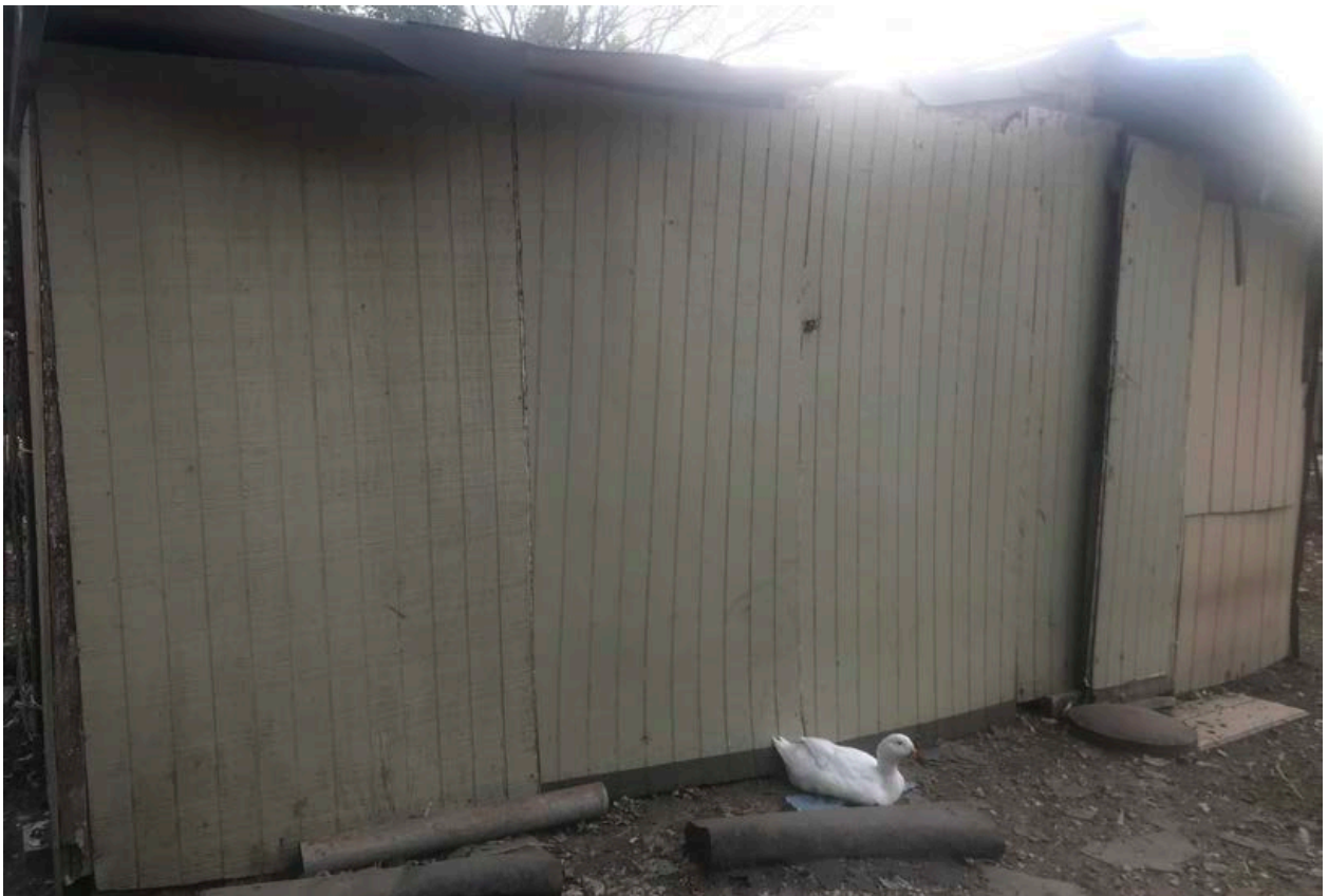
Figure 5. Photograph of an accessory structure at 3740 North 35th Street (provided by the applicant).
