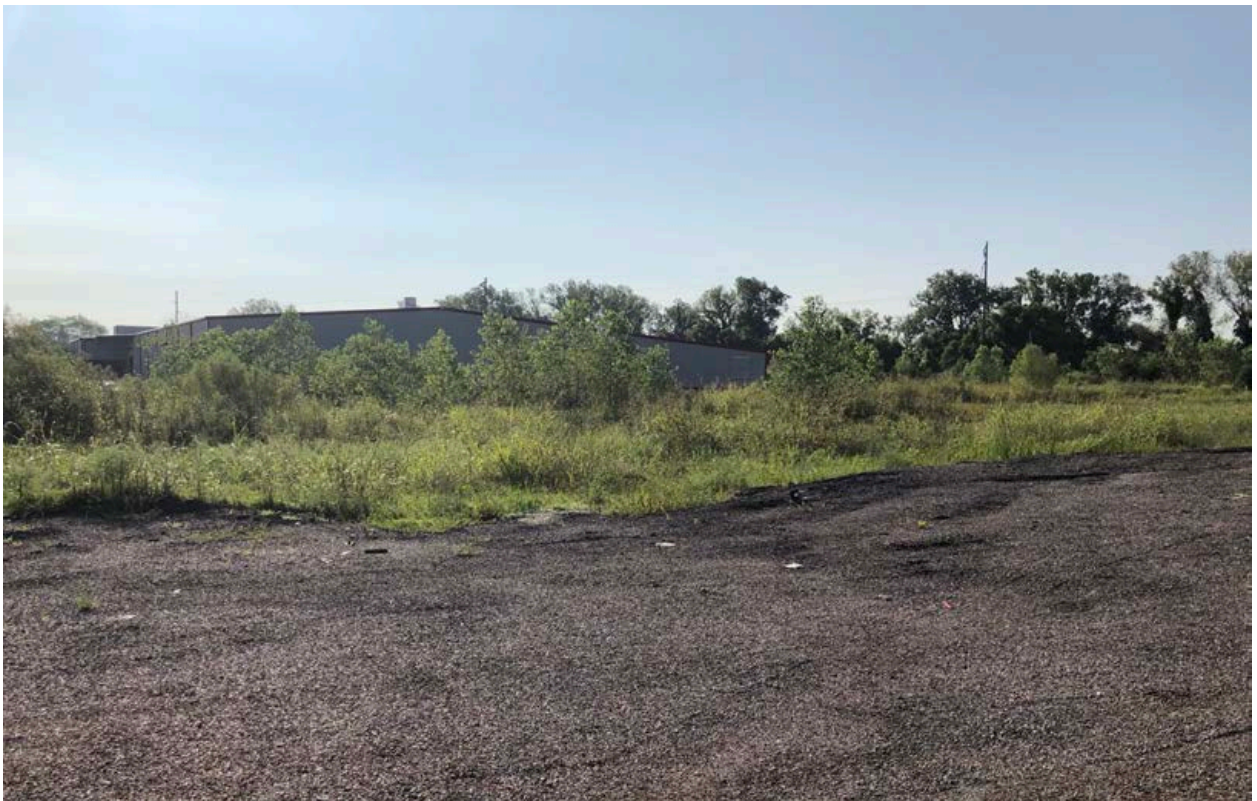
Figure 5. Figure 4. Site Photograph of 1625 South 86th Street looking southeast (provided by Planning Staff).
