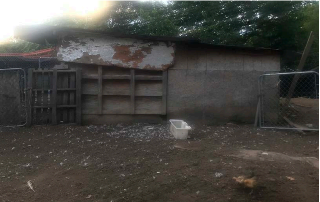
Figure 7. Photograph of an accessory structure at 3740 North 35th Street (provided by the applicant).
