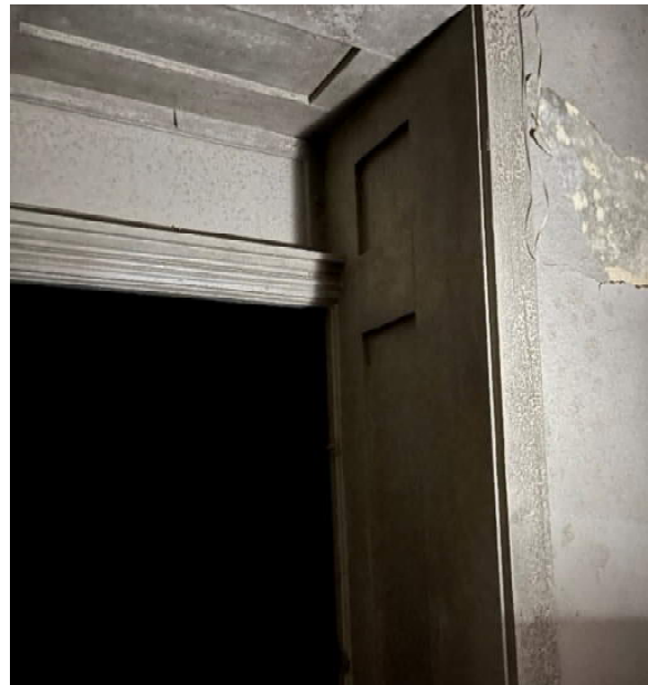
Image 21 – Paneled jamb casing, lower level (1 of 1).
