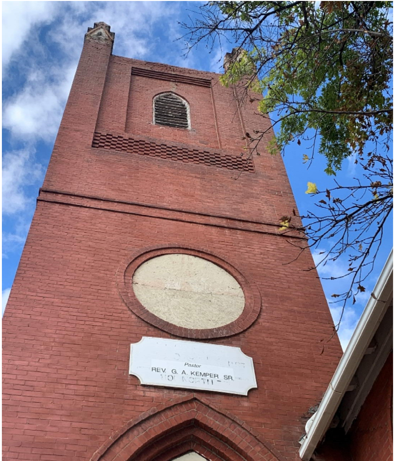
Image 10 – Bell tower with ornamental metal engaged pier cap.
