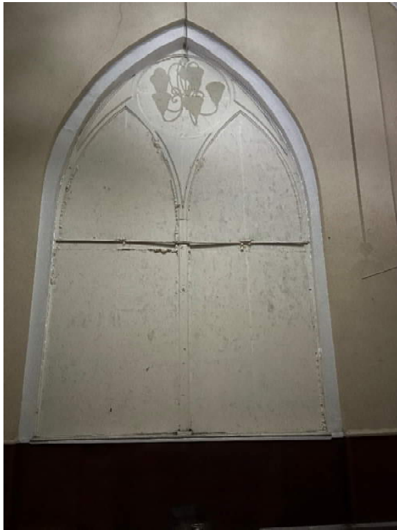
Image 1 (Left) – Center stained-glass windows in worship area (2 of 2); these windows should be further investigated by removing the plywood to determine if they are for candidates for salvage. Image 2 (Right) – Typical worship area stained-glass windows (6 of 8).
