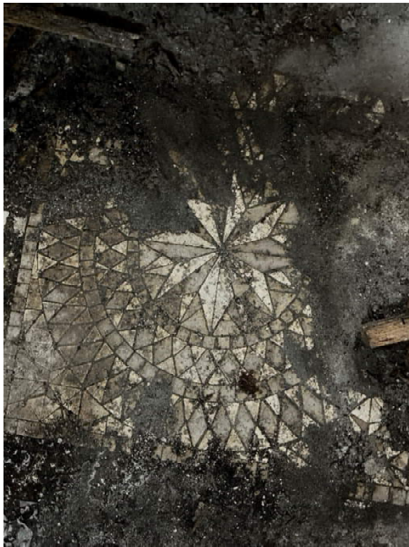
Image 26 – Encaustic floor tile in main foyer.
