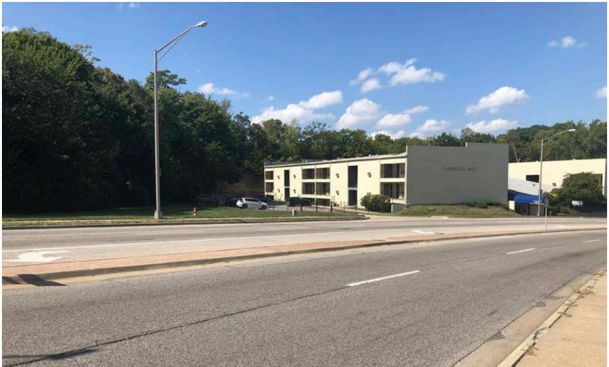
Figure 7. Site Photograph of 3600 Rainbow Boulevard looking northeast (provided by Planning Staff).
