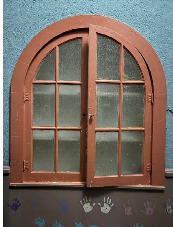
Image 25 – Built-in casework with glass doors (1 of 2).
