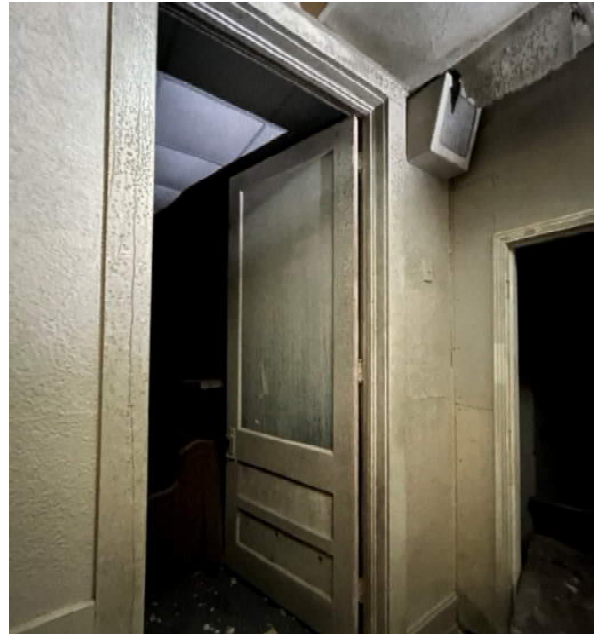
Image 14 (Left) – 5-paneled swinging doors at base of stair (1 of 1). Image 15 (Right) – 2-paneled doors with lights into classrooms (8 of 8).
