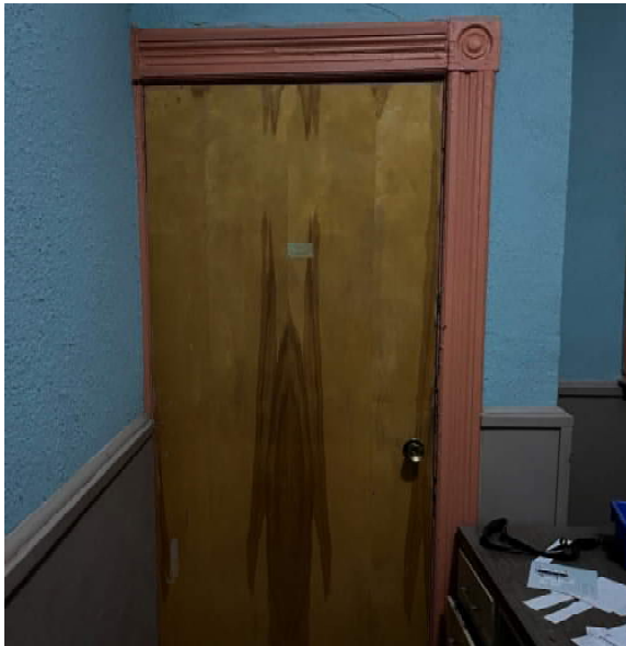
Image 18 and Image 19– Typical molded door and windows casings with bullseye rosettes.
