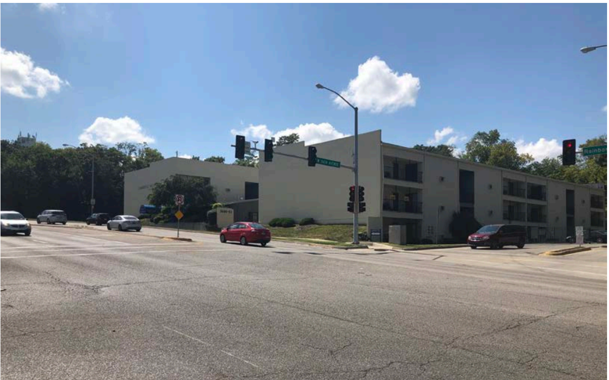
Figure 5. Site Photograph of 3600 Rainbow Boulevard looking northwest (provided by Planning Staff).
