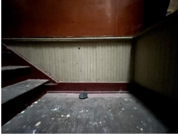
Image 22 – Beadboard wainscot and wood base at stair.
