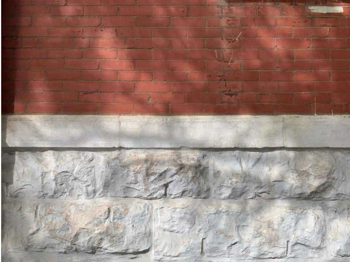
Image 9 – Typical red brick, tooled limestone water table course, and rough-cut limestone foundation.
