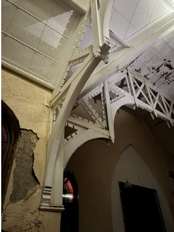
Image 28 and Image 29 – Ornamental wood trusses in main worship area.
