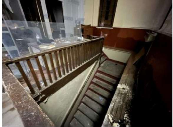
Image 23 – Wood guardrail at stair.
