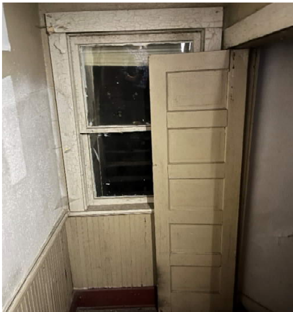
Image 20 – Typical flat window and door casings.
