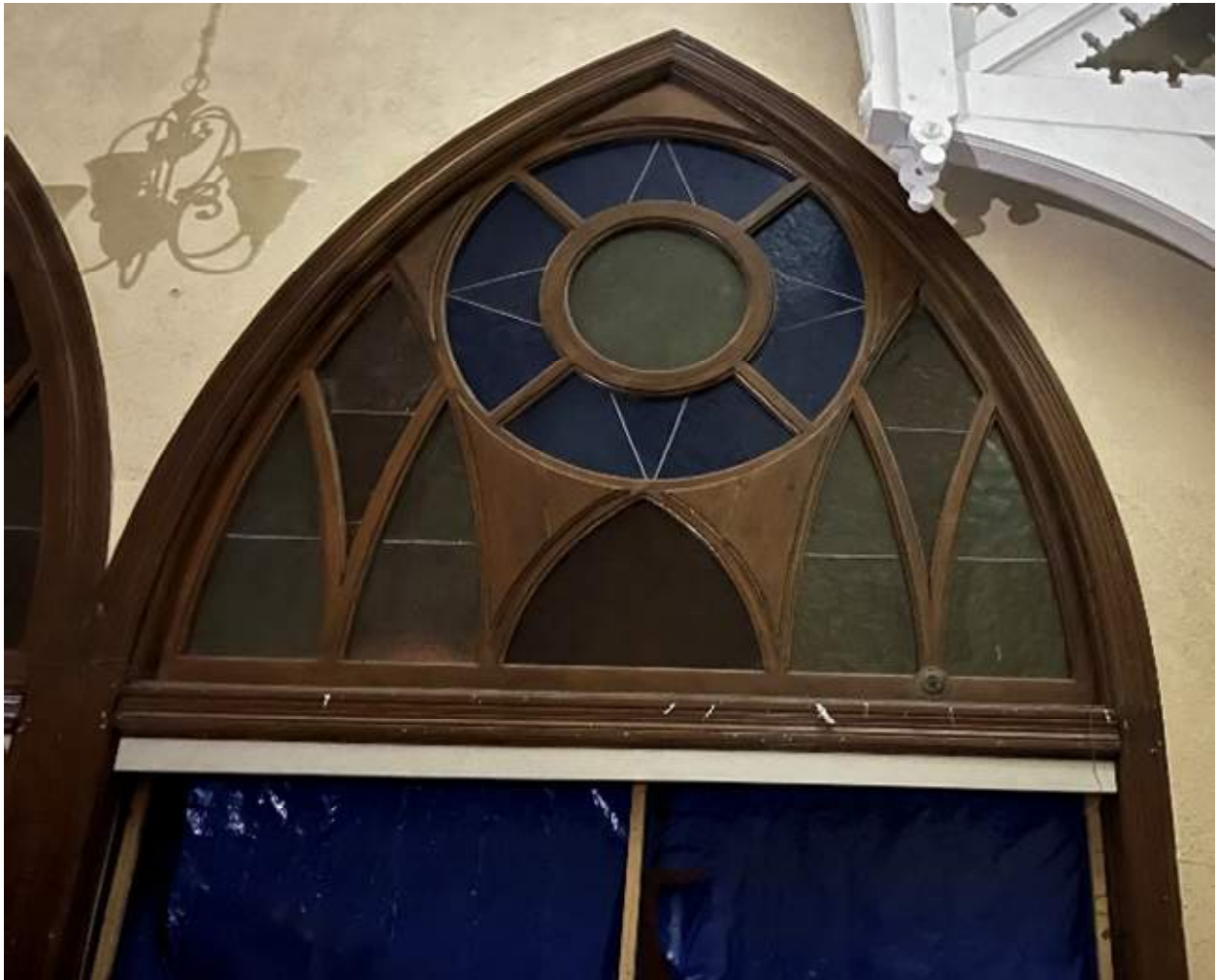
Image 11 – Stained-glass pointed-arch transom windows at openings between narthex and worship area (3 of 3).
