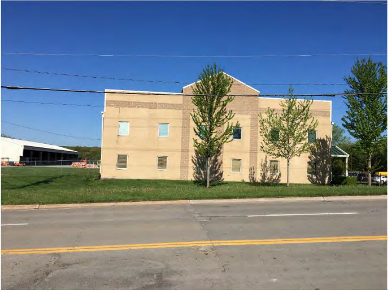
Looking west from 47 th Street – existing office/warehouse building, equipment storage building in background
