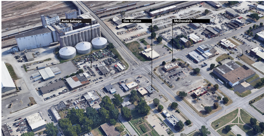
Above: View of the Intersection of 7th Street and Kansas Avenue, Facing West (PORT) Below: Aerial View of the Intersection of 7th Street and Kansas Avenue (Google Earth)
