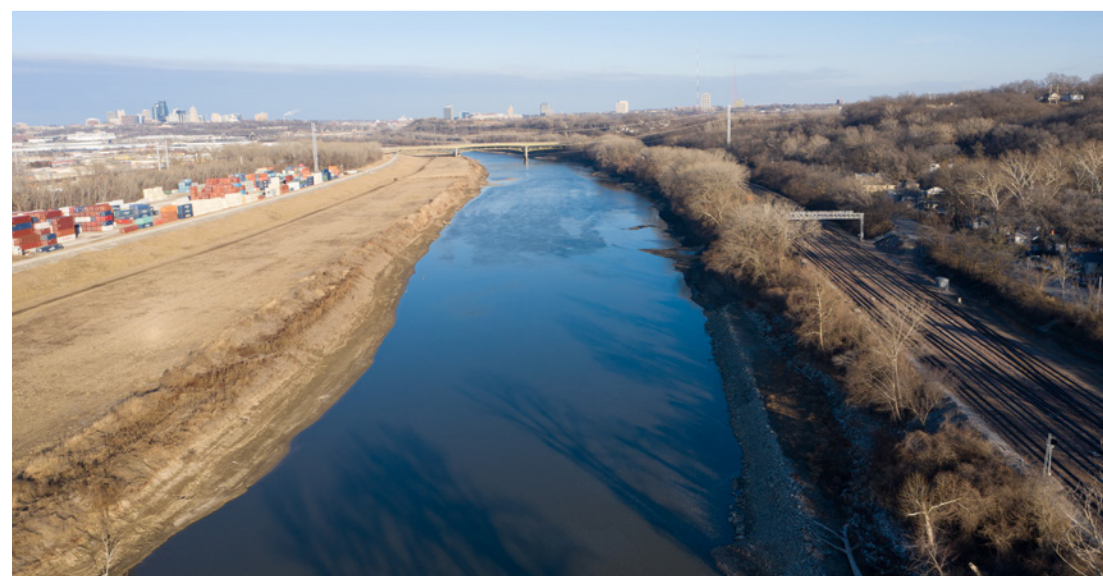
Above: Aerial Photo of Armourdale and the Kansas River, Facing East (PORT)
