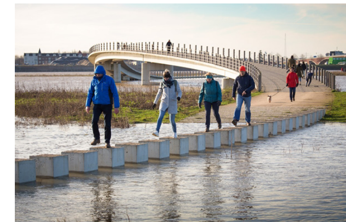
Room for the River, The Netherlands: more space for rivers, while adding leisure facilities and connections to riverfront communities.
