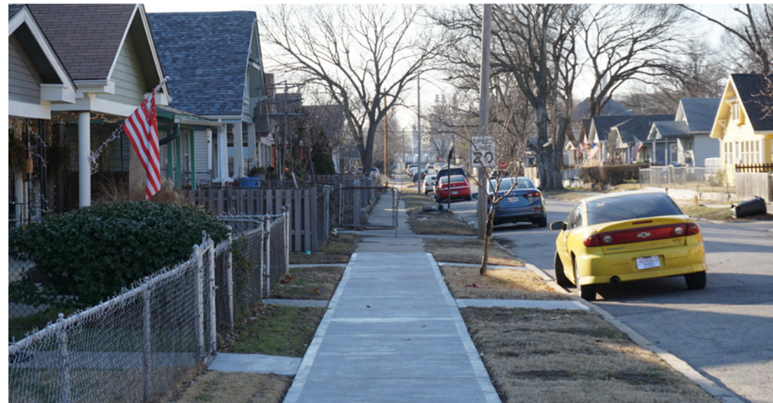
Above Top: Neglected Public Sidewalks (PORT)
