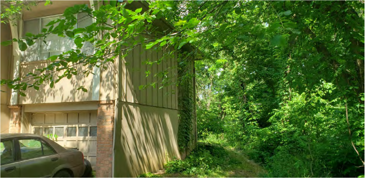
Figure 9. Site Photograph of 609 – 611 South 75 th Street (provided by the applicant).
