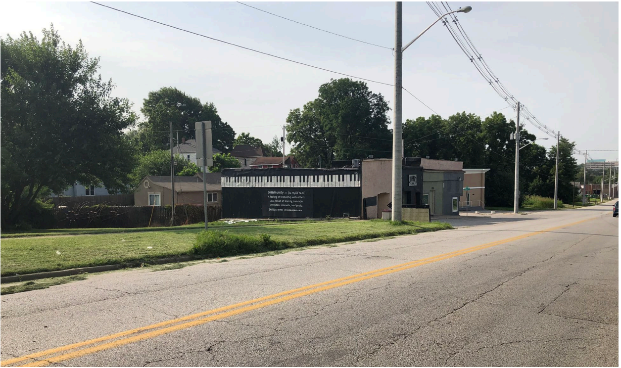
Figure 6. Site Photograph of 2005 North Thompson Street (provided by Staff).
