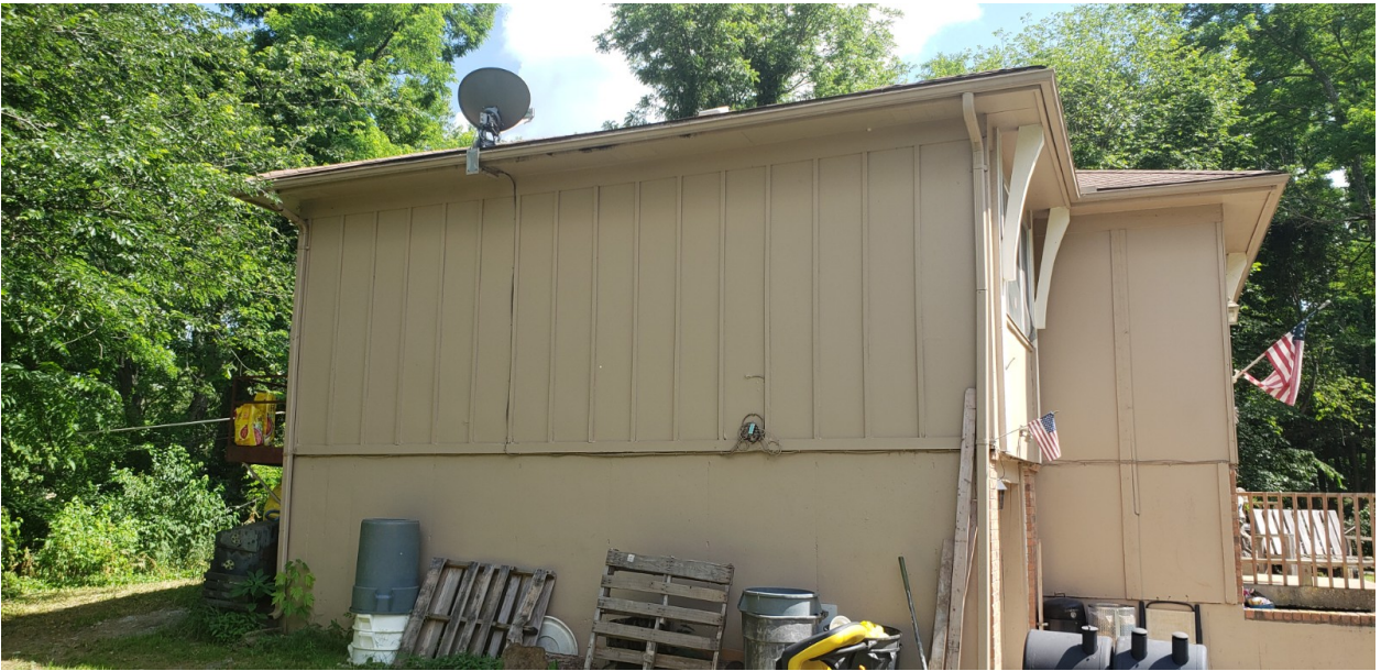
Figure 8. Site Photograph of 617 – 619 South 75 th Street (provided by the applicant).
