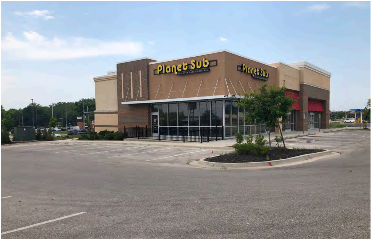
Figure 4. Site Photograph of 7750 State Avenue looking southwest (provided by Staff).
