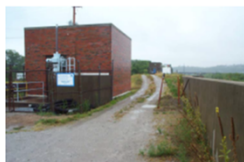
Osage Avenue Pump Station (Armourdale)
