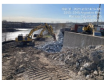
Argentine Main Pump Station Demolition
