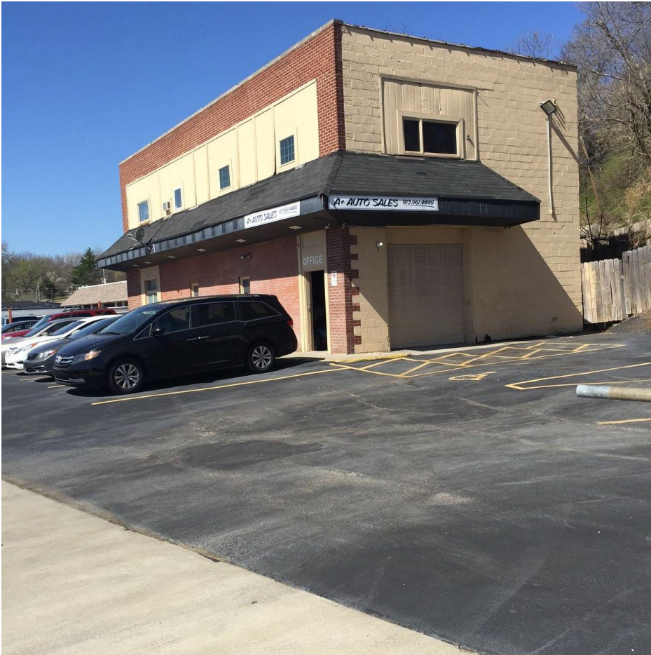
Figure 6. Site Photograph of 1010 Merriam Lane taken on March 30, 2021.
