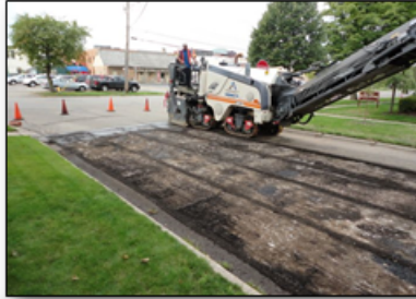
Above: Street milling operation. First step needed in resurfacing projects.
