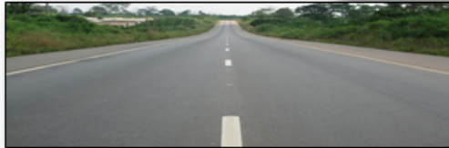
Left: View of freshly paved and marked road.
