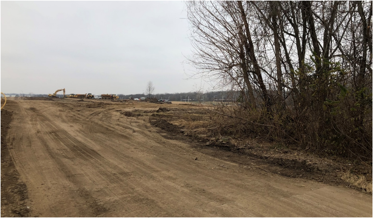
Figure 6. Site photograph on North 69th Street looking southeast at Turner Logistics Center (provided by Planning Staff).
