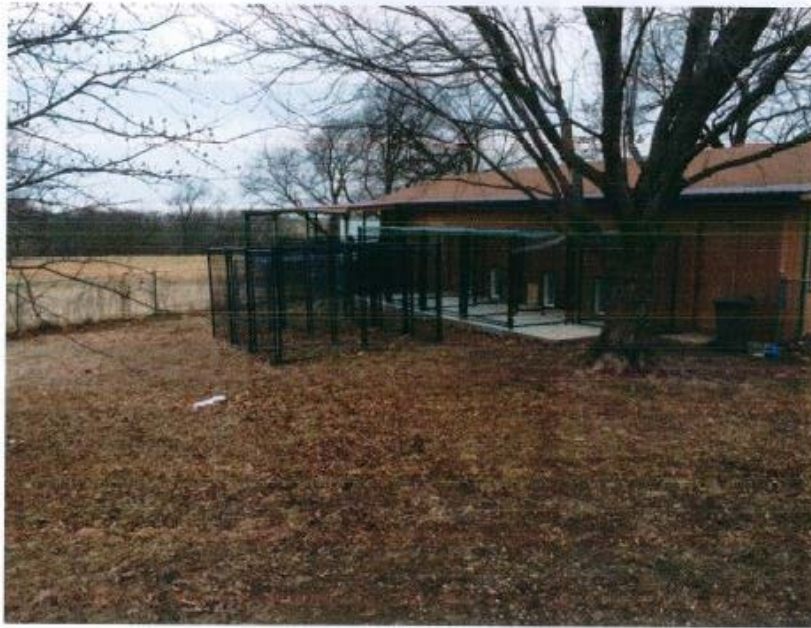
Outside Runs & Yard
