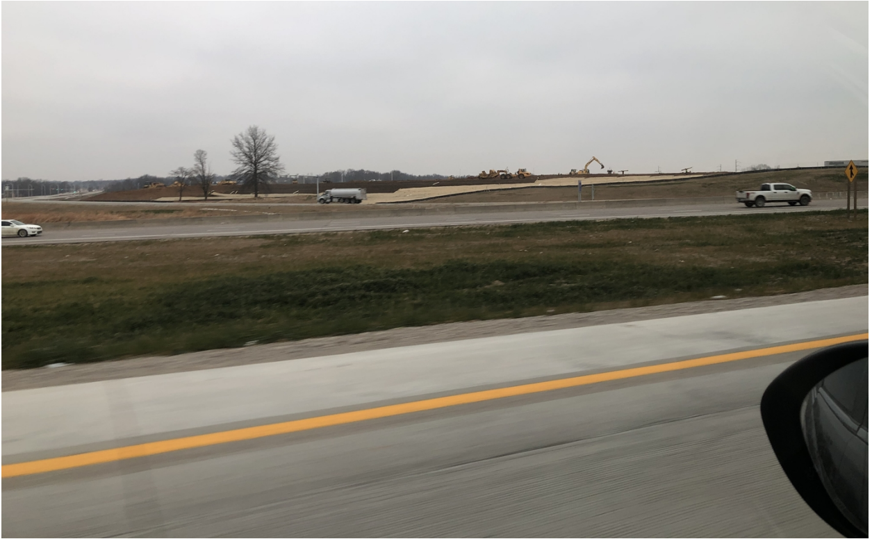
Figure 6. Site photograph of Turner Logistics Center looking north on I-70 East ramp (provided by Planning Staff).
