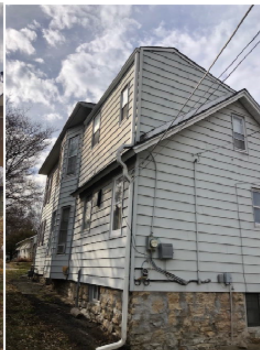
NE Corner of back of duplex
