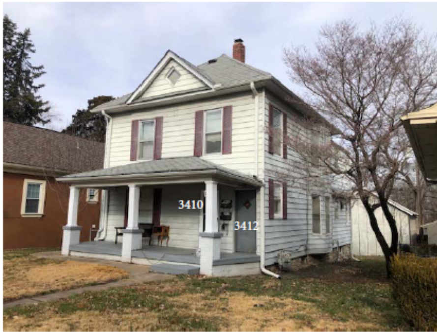
SE side of front of duplex. Facing Metropolitan Ave.
