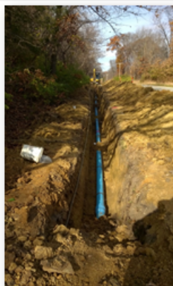
Above: Construction of the Wyandotte County Lake Waterline.
