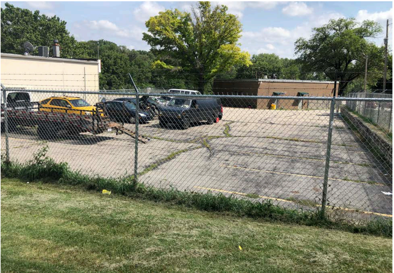
Figure 4. Site photograph of the parking lot at 2120 Park Drive (provided by Planning Staff).
