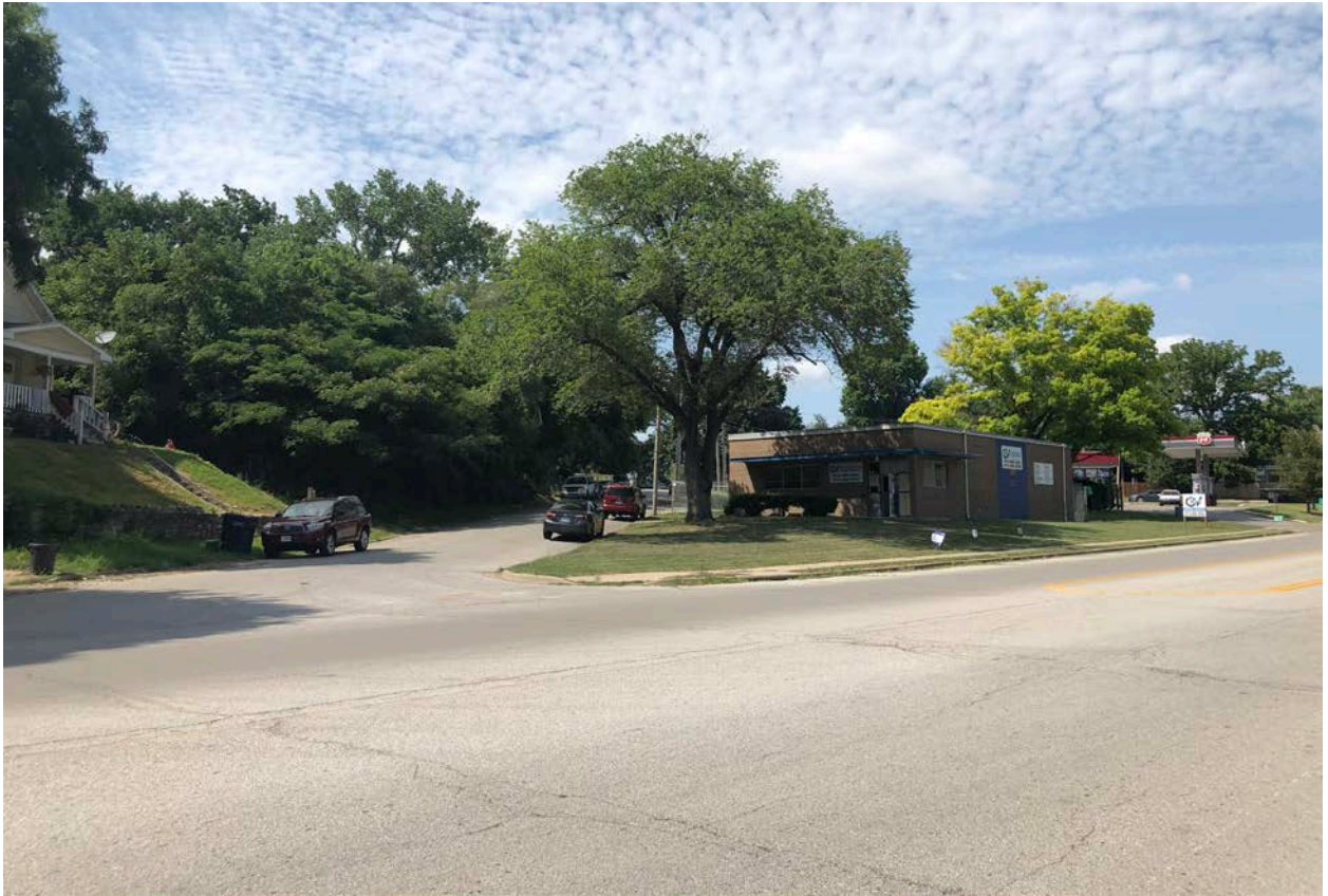
Figure 1. Site photograph of 2120 Park Drive looking north (provided by Planning Staff).
