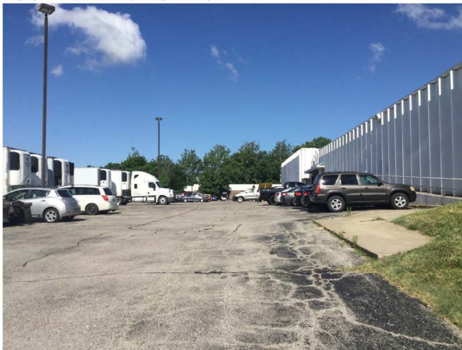
Staging to the left addition parking to the right
