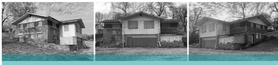
The historic Parks and Rec building in Clifton Park
