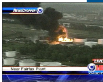
One of the fuel tanks in Fairfax on fire on June 4, 2008 after it was struck by lightning (courtesy KIMB-TV)
