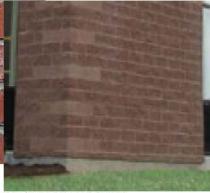
SPLIT FACE MASONRY BLOCK - BUFF / TAN
