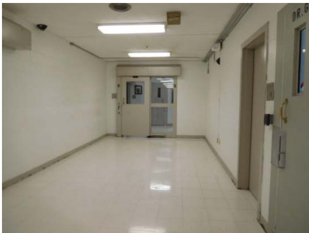
Typical corridor in detention area
