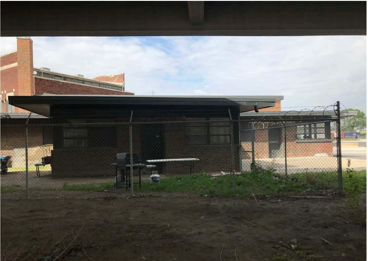
Figure 4. Photograph of the side of the building looking north (provided by the applicant).
