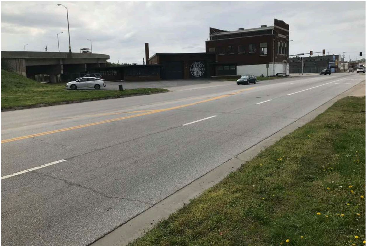
Figure 2. Photograph of the parking lot and building looking northwest (provided by the applicant).
