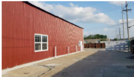
Back of the building
