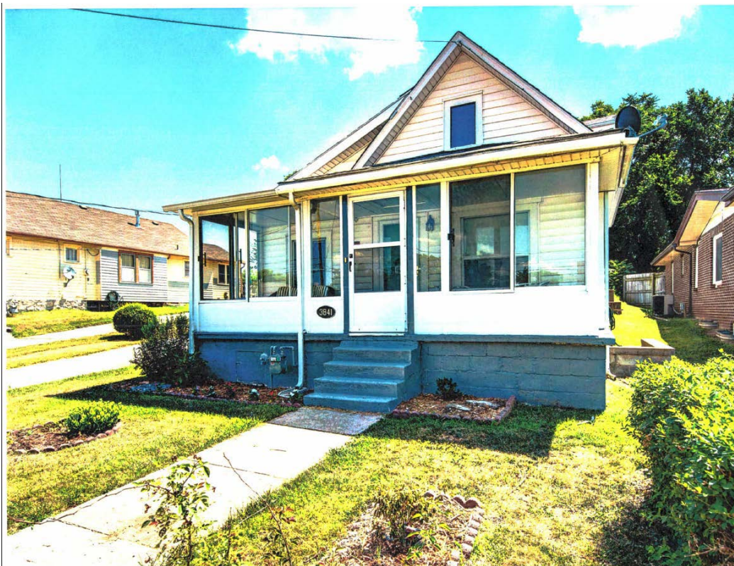
Figure 2. Photograph of 3841 Lloyd Street (provided by the applicant).
