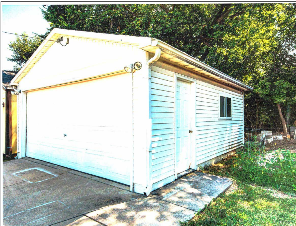
Figure 9. Photograph of the two-car garage at 3841 Lloyd Street (provided by the applicant).
